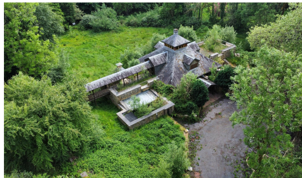
The former restaurant building (DM Auctions, 2024)
