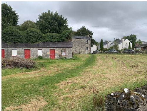
A desire line path from the town centre to the Depot CS observed during the survey
