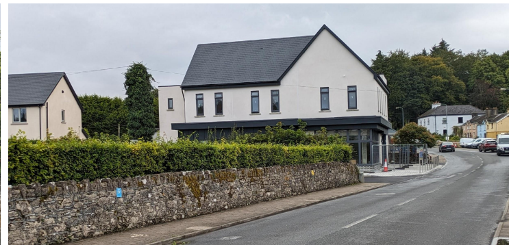
New library building
