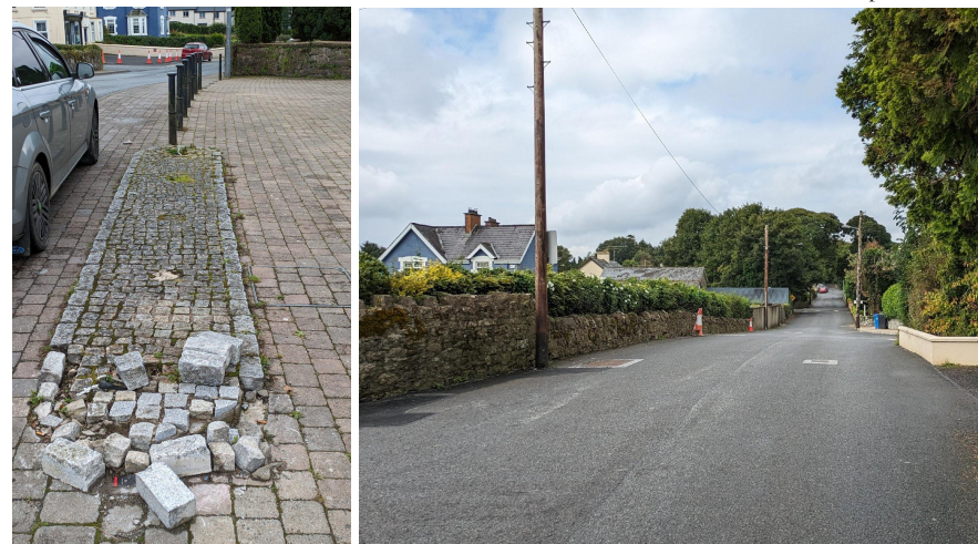
Observed during the study visit, obstructions on pavements on Mains Street and the lack of dedicated pavements of Back Line
