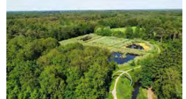
Lankheet Water Purification Park, The Netherlands
