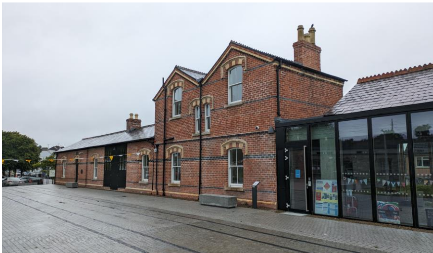
The Junction Hub
