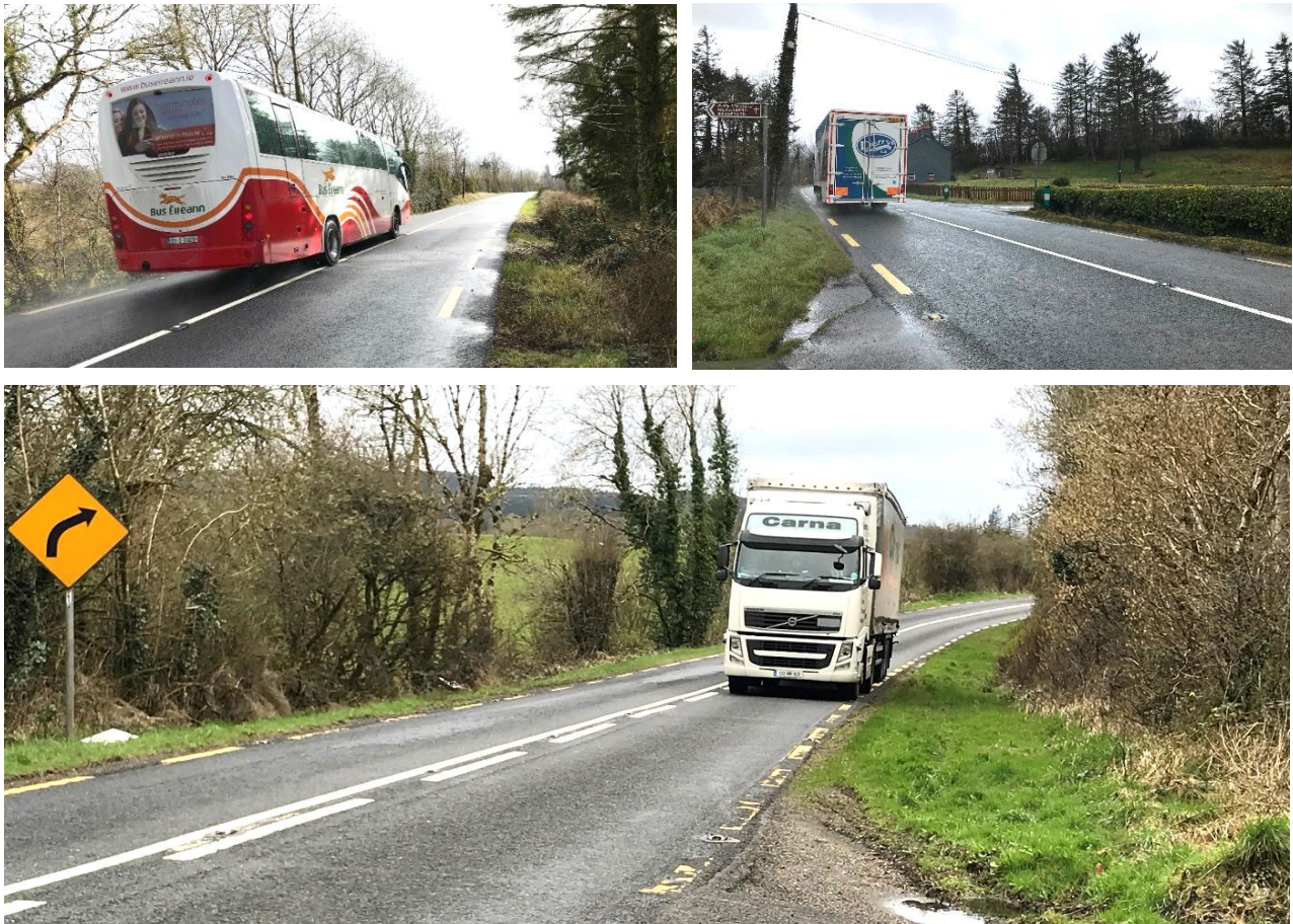
Figure 2-2: Photographs of the existing substandard N16 cross section
