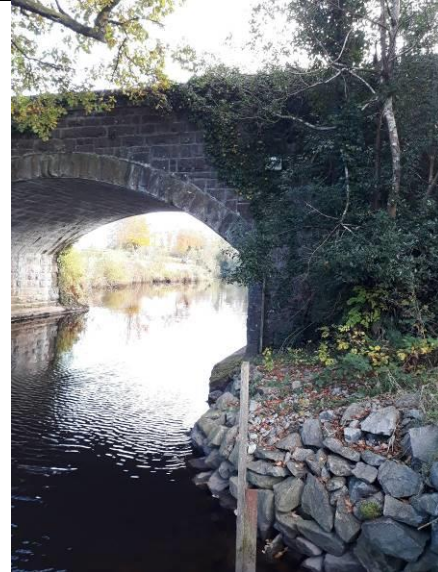
Plate 2 Aghoo Bridge, the pedestrian underpass will be connected to the right side of the bridge arch, as viewed from this image.
