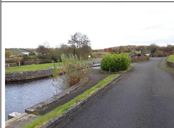
Plate 11 View of the existing facilities at Lock 4, the eastern terminal end of the proposed development.
