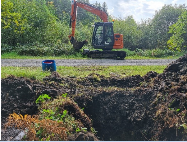
Facing East From the Trial Hole Excavation
