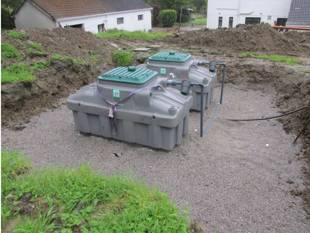
Photograph – Example of Ecoflo Co co Filter Under Construction
