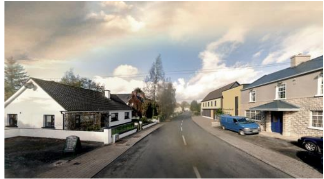
Existing/Proposed View –facing North West
