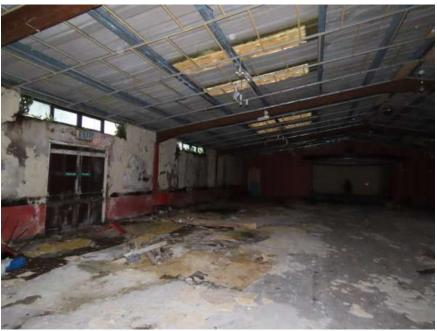
Photo 7 – dance hall building with asbestos roof
