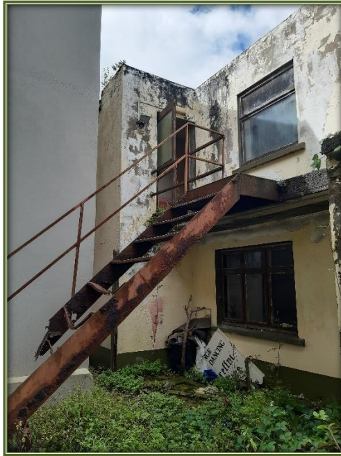
Plate 1 – Building at the Back of the Site
