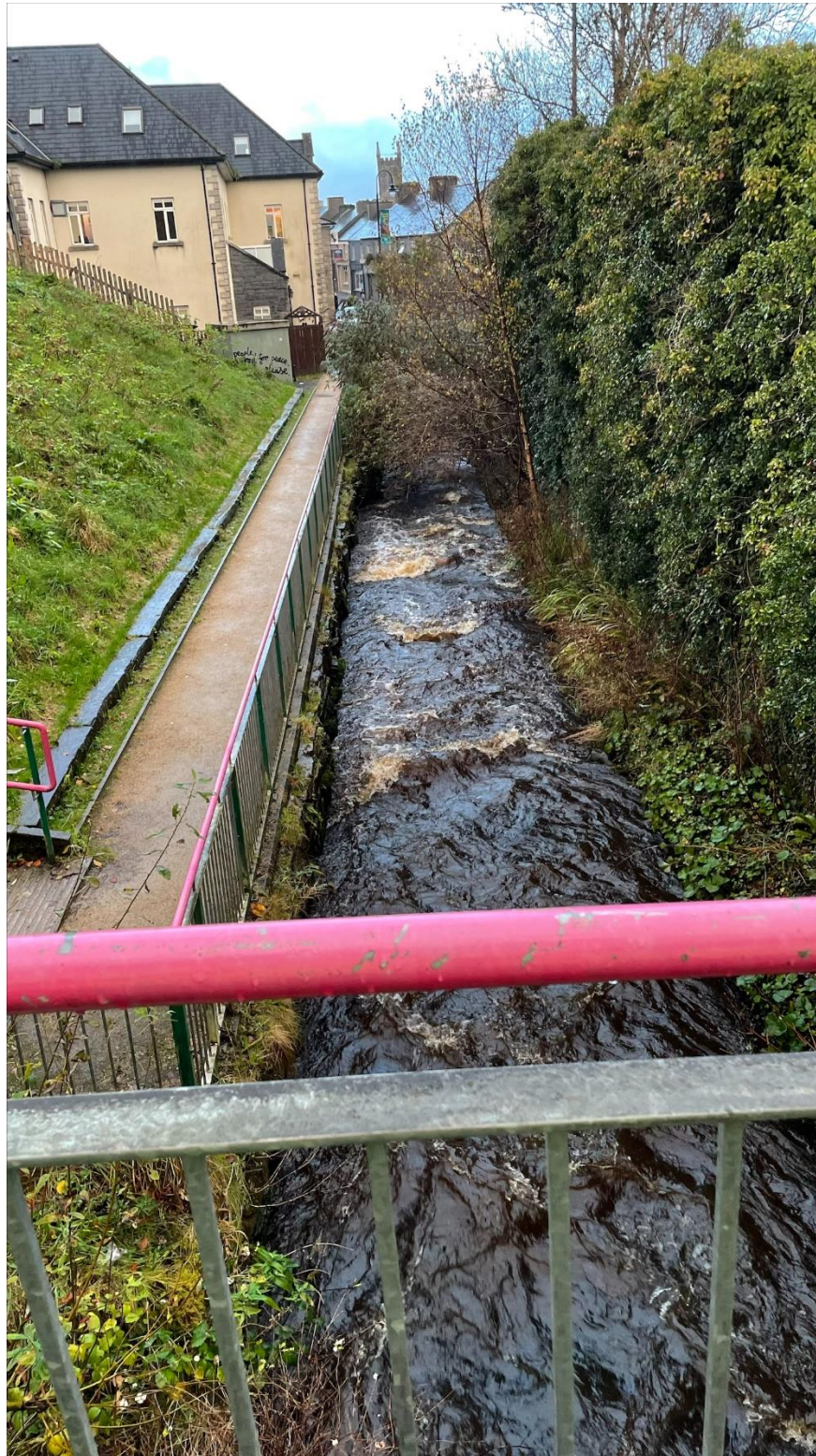
Image 4: B3 (Image taken from steel bridge, facing northwards)
