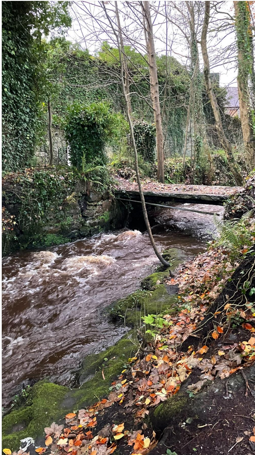
Image 3: B2 (Image taken from west embankment)
