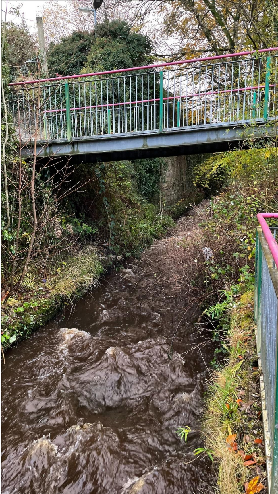
Image 5: B3 (Image taken from steel bridge, facing southwards)
