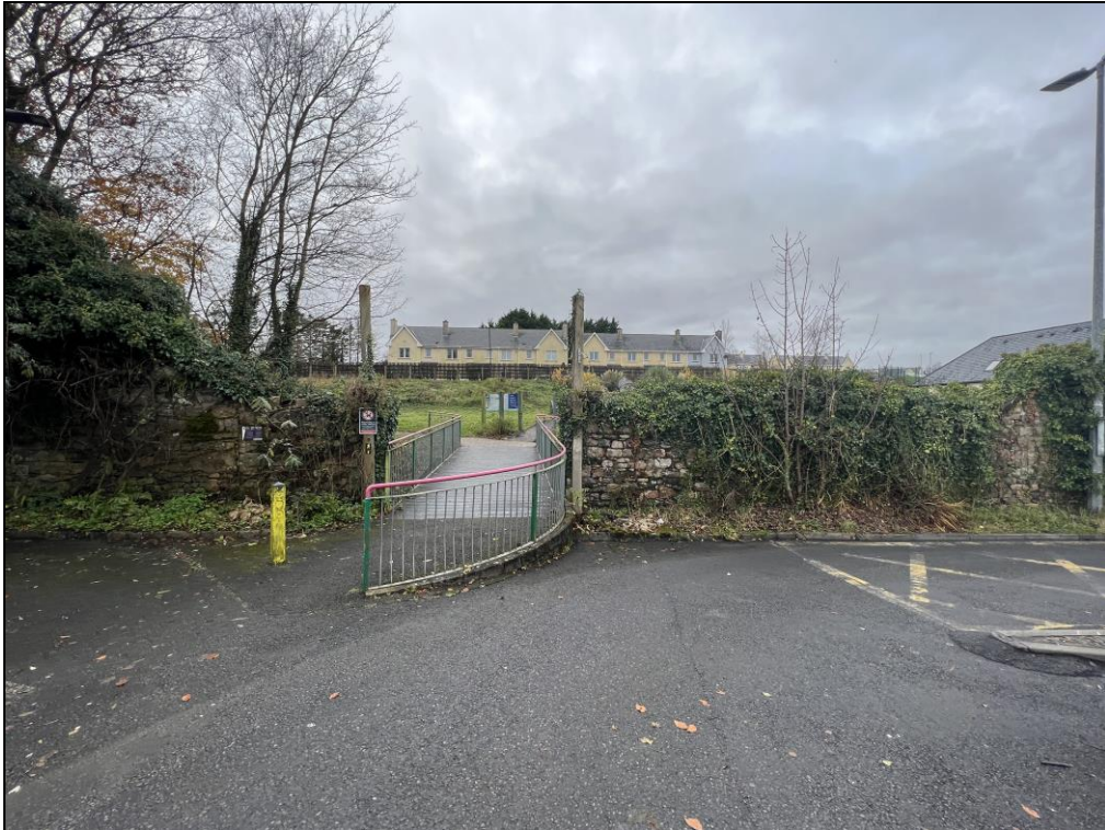
Plate 2: West facing view of the existing bridge and access to the People's Park from Market Yard.
