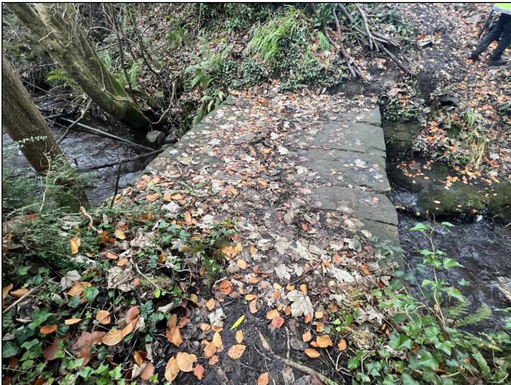
Plate 9: Detail of the stone flagged bridge.
