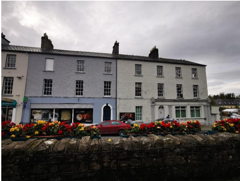
Figure 3. Photograph - Existing Buildings along Main Street
