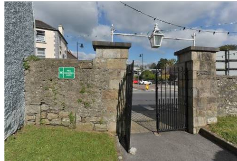
PIC. 3; ENTRANCE (FROM WITHIN)
