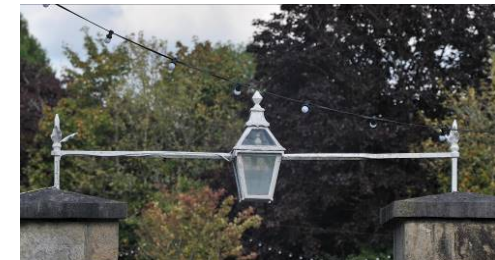
PIC. 5; WROUGHT/CAST IRON LANTERN OVER ENTRANCE.
