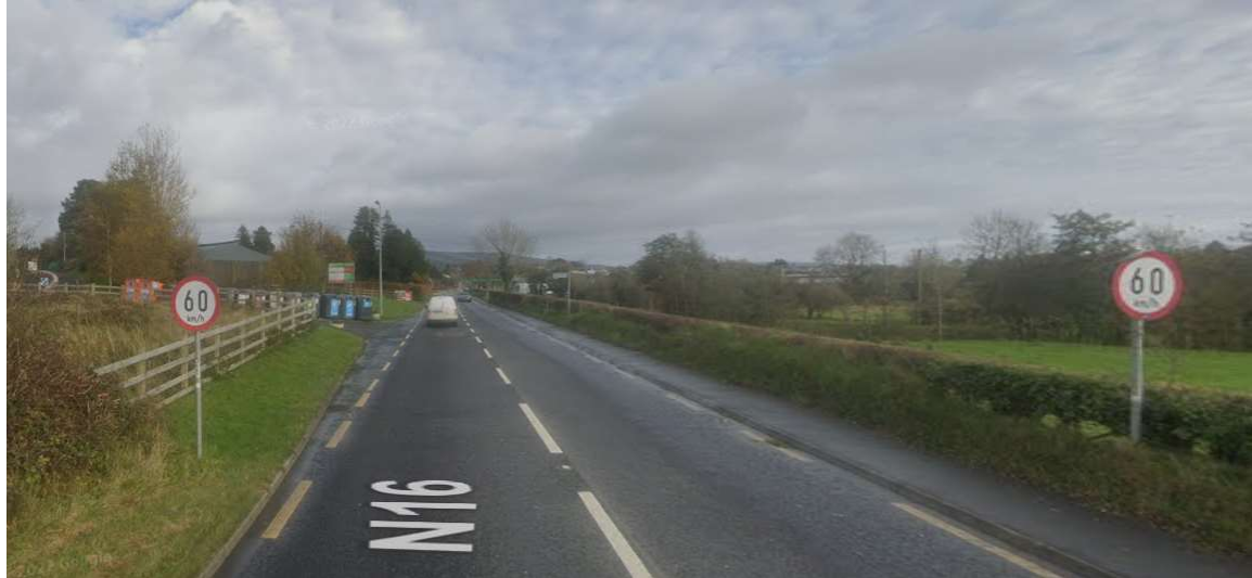
Figure 3: Existing restricted speed limit along roadside frontage of proposed Fire Station site (Source: Google Streetview, November 2022)
