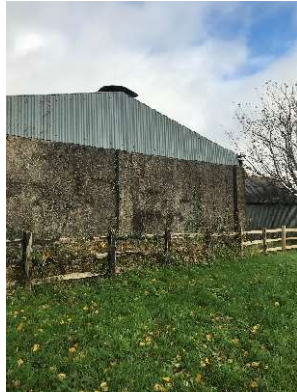
Shed Adjacent to Site
