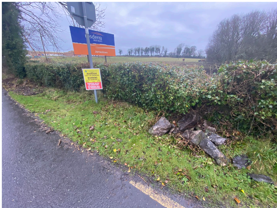
Plate 1: NW facing view of the stone wall field boundary at the eastern end of the proposed footpath
