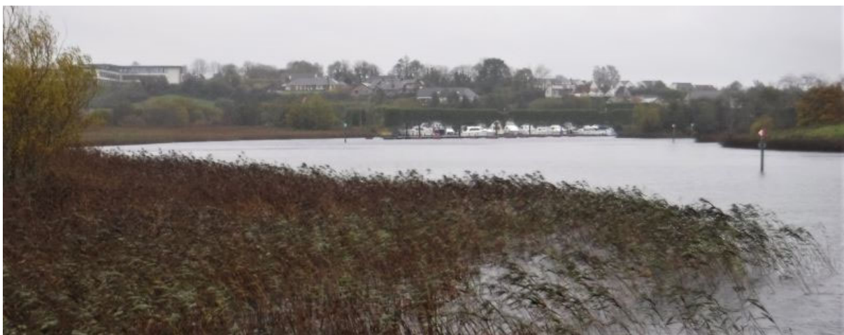
Photo 20: View East of River Shannon. The drainage channel enters the river near the boat marina.
