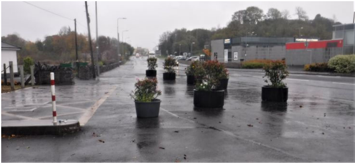
Photo 18: View East of the N4 where the drainage channel is culverted into the Carrick Retail Park.
