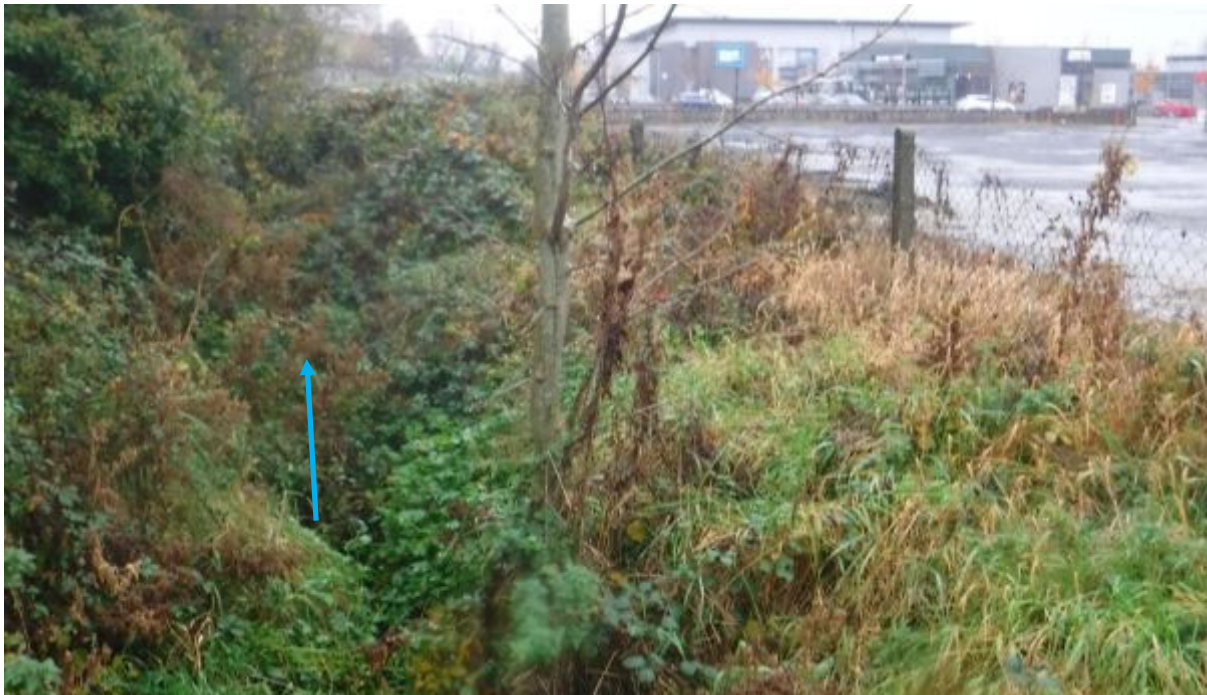
Photo 16: View South of open channel which flows beside the GAA carpark area.
