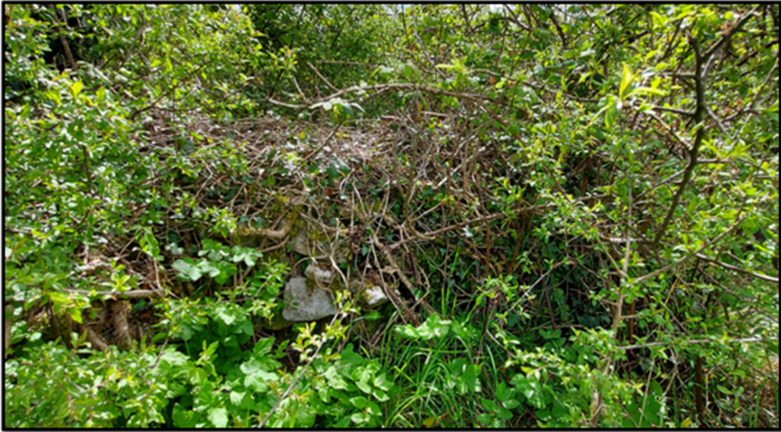
Plate 3.2 Stone wall with dense entangled vegetation.
