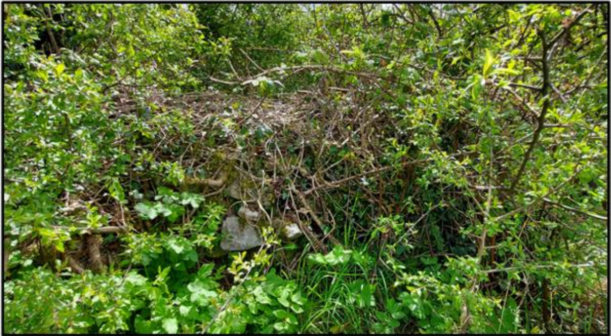
Plate 2.2 Stone wall with dense entangled vegetation.
