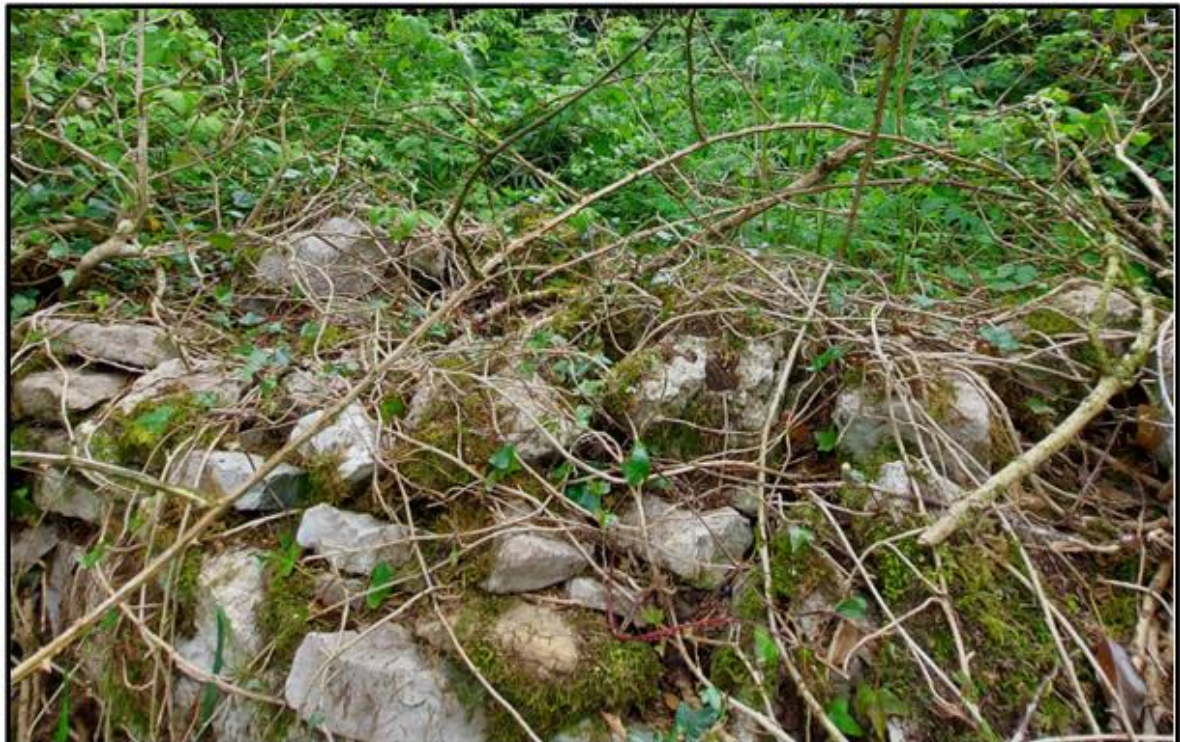
Plate 2.3 Stone wall along the walking/cycling greenway recreational trail northwestern boundary.
