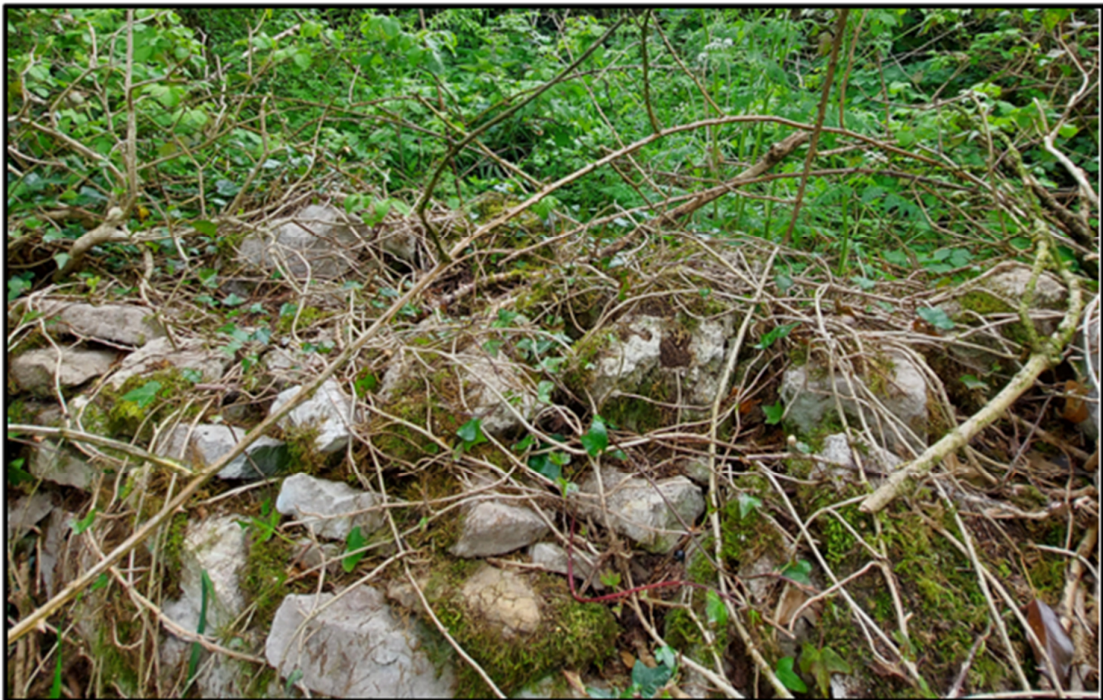
Plate 3.3 Stone wall along the northwestern boundary.
