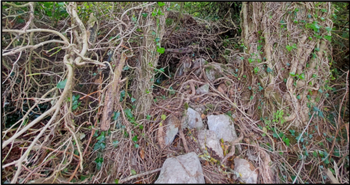
Plate 3.4 Collapsed stone wall showing densely entwined ivy vines
