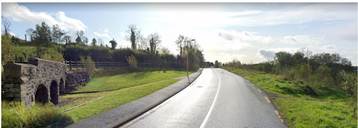
Figure 4: View of the triple arch bridge on the Convent Avenue which will be the crossing point The Greenway will pass through the central arch of the bridge.
