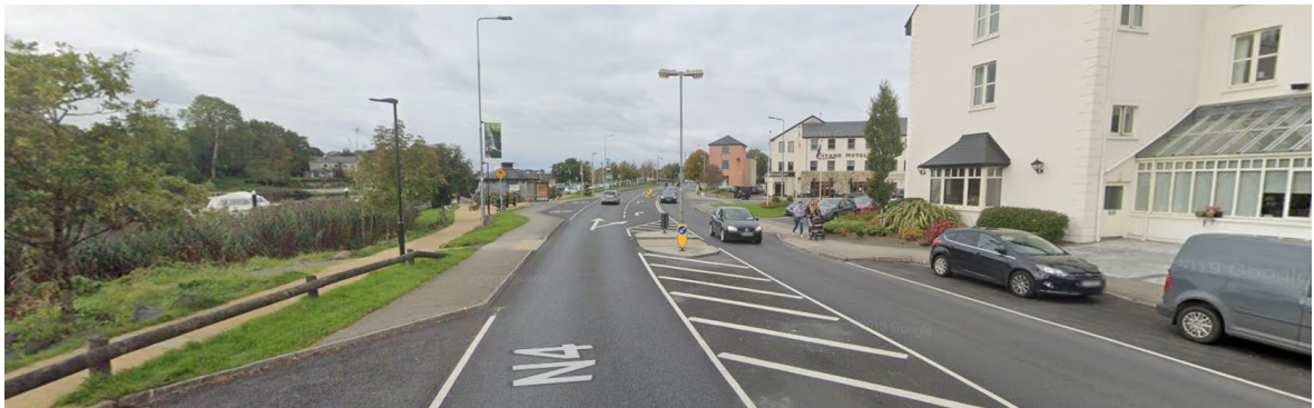
Figure 1.2: A view of the scheme from the N4 east of the junction
