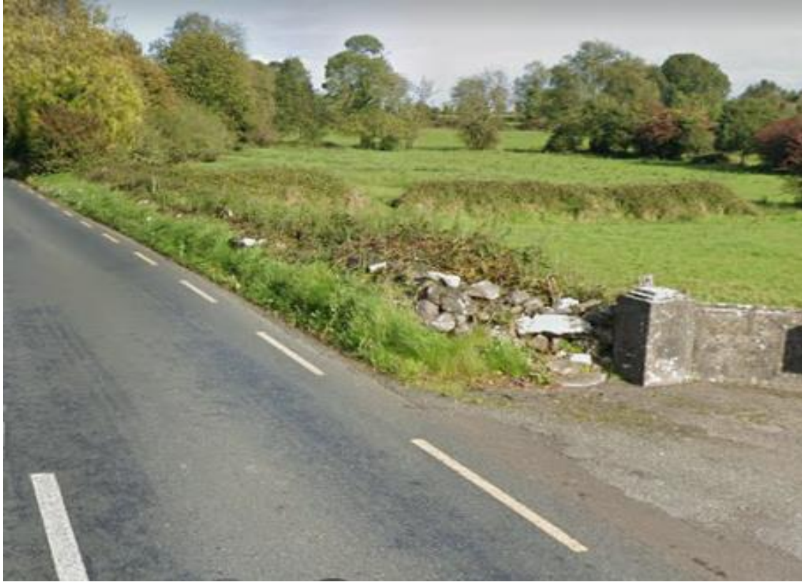
Photo #1: Location of proposed new 55m greenway section east of the R-209.
