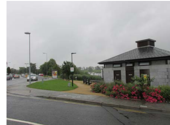
View of current public toilets with bus stop in background
