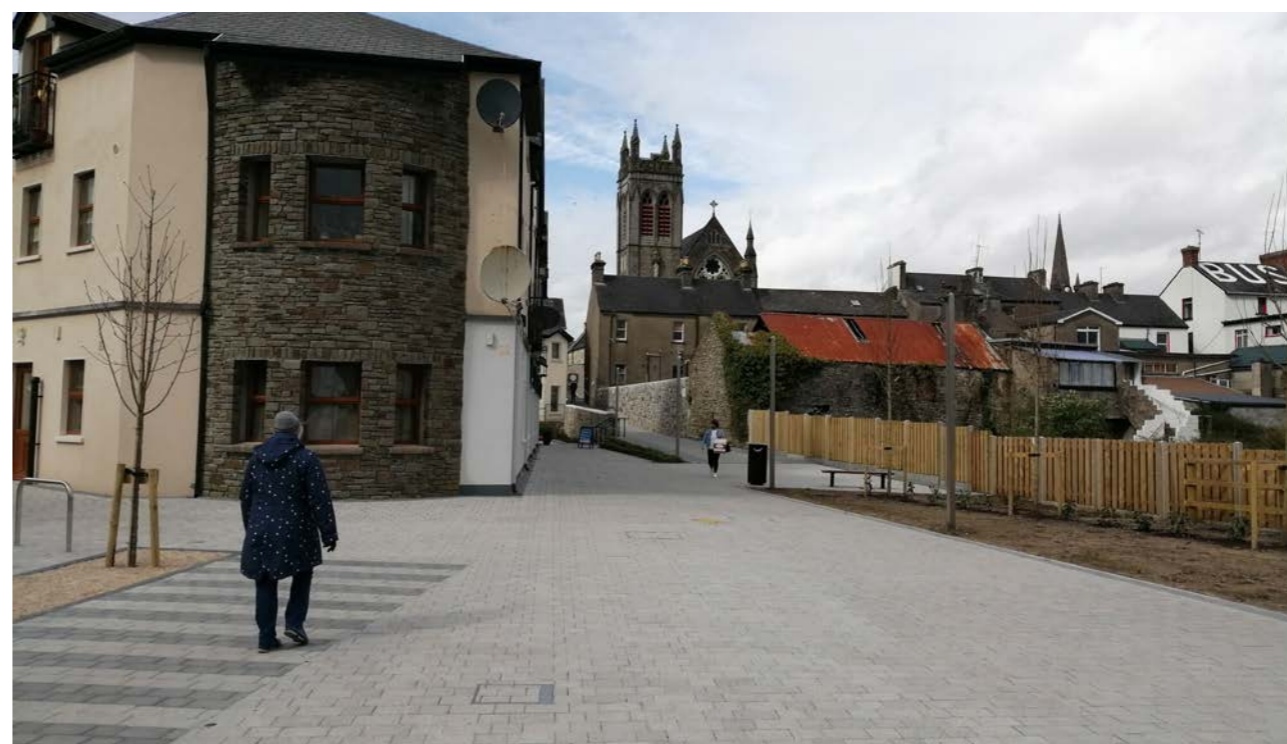
Block paving product made with sparkling granite aggregates, Flynn's Field To Footpath
