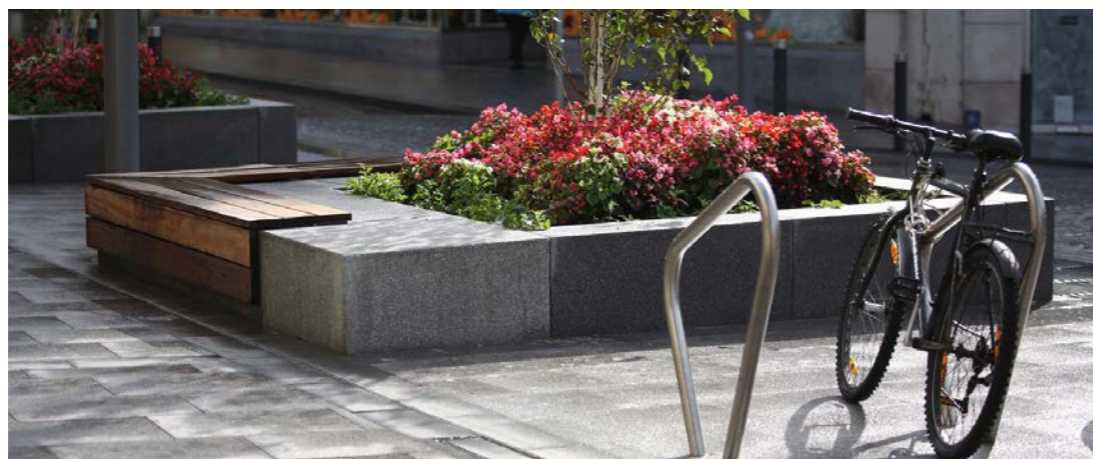
Wooden Bench on Concrete/stone block To Seating areas
