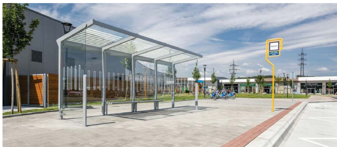
BUS Stop with gantry structure and glass roof
