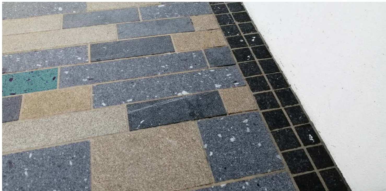
Existing materials palette and colours from public realm improvement scheme.
