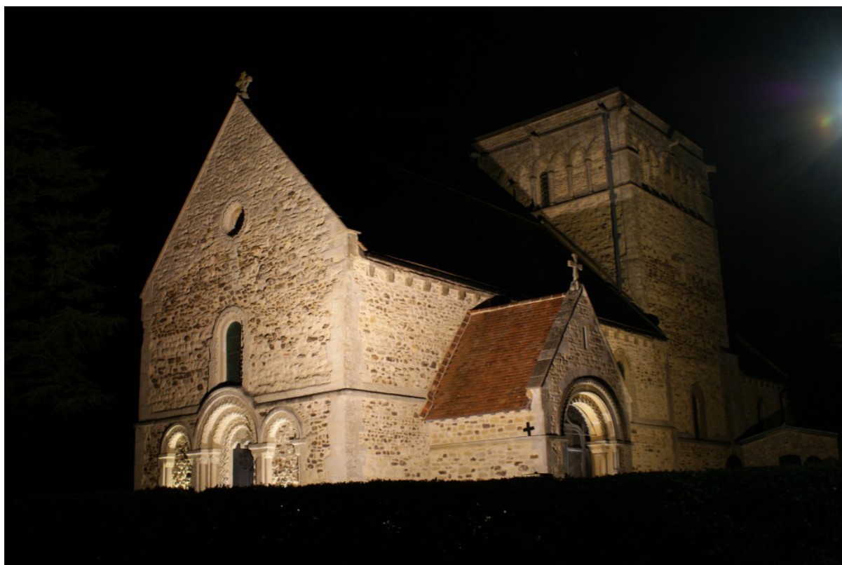
Example of warm LED lighting on stone church facades
