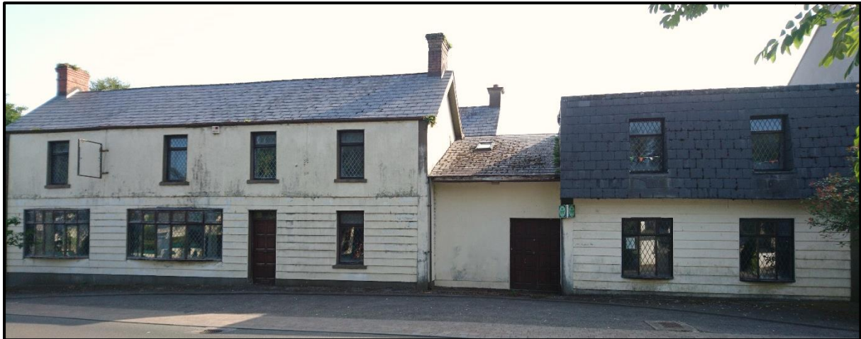
Plate 2: View of the site looking eastwards from the opposite side of Main Street
