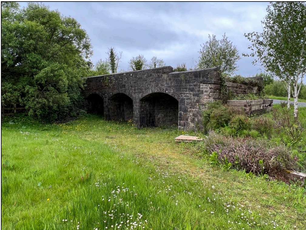
Plate 4: SW facing view of the railway bridge at Chapel Street.
