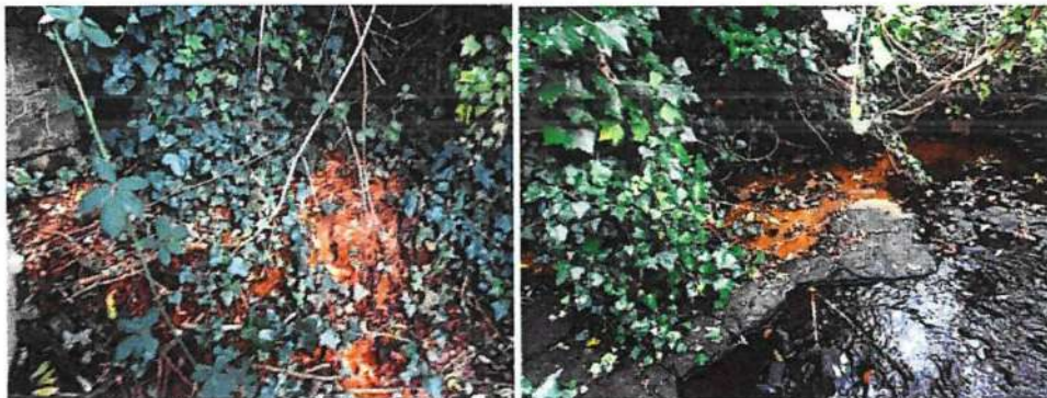
Figure 4: Landfill Discharge Box Culvert
