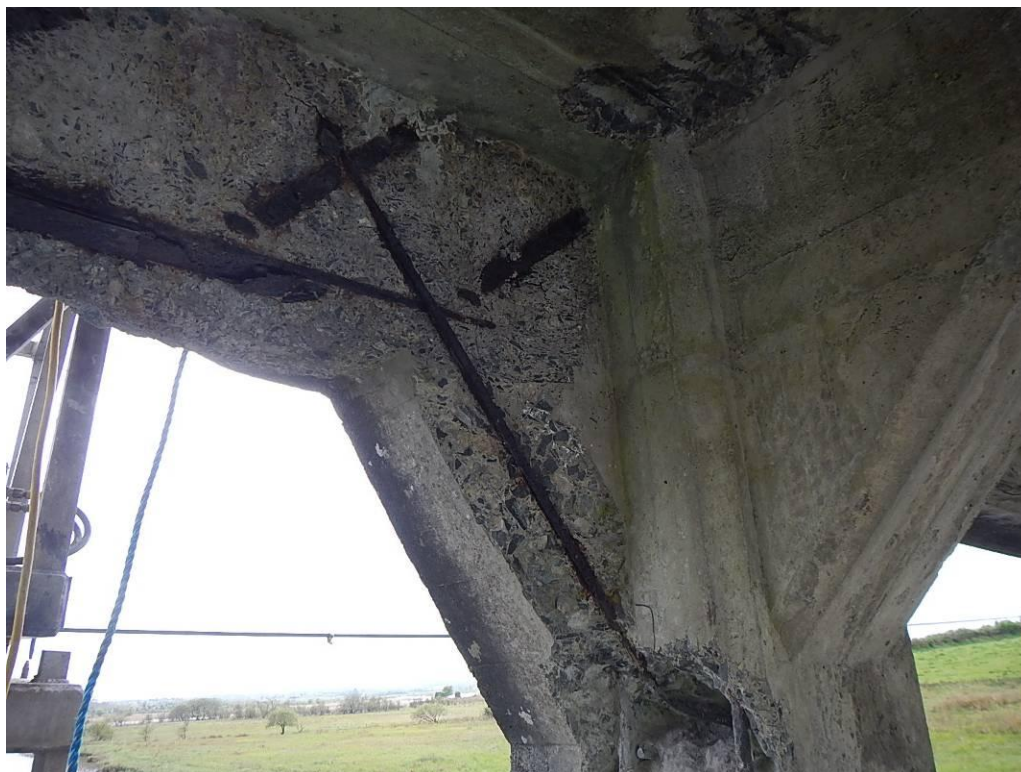
Photograph 13: Bridge Beam Span 3 / Pier 3 South
