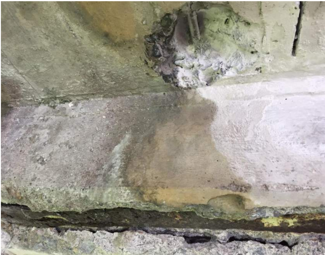
Breakout to confirm transverse reinforcement
