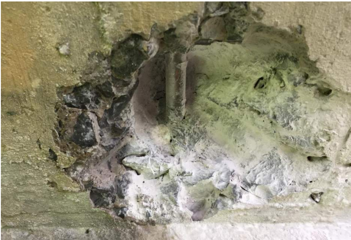
Close up of transverse reinforcement
