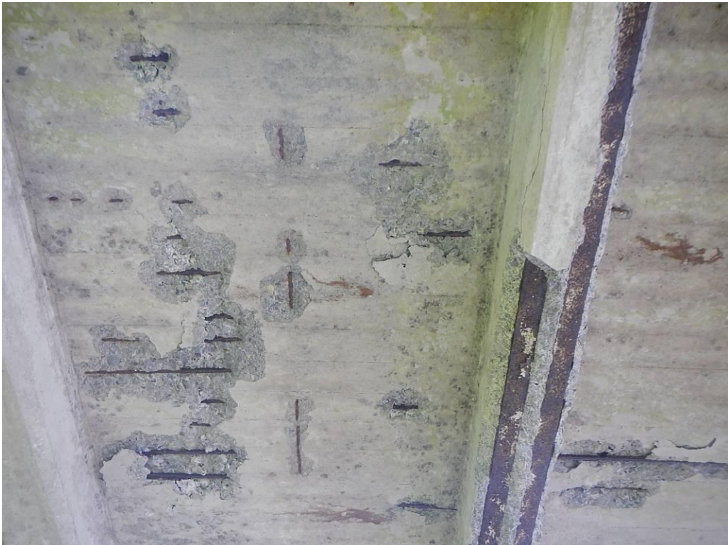
Photograph 10: Bridge Deck –Span 6
