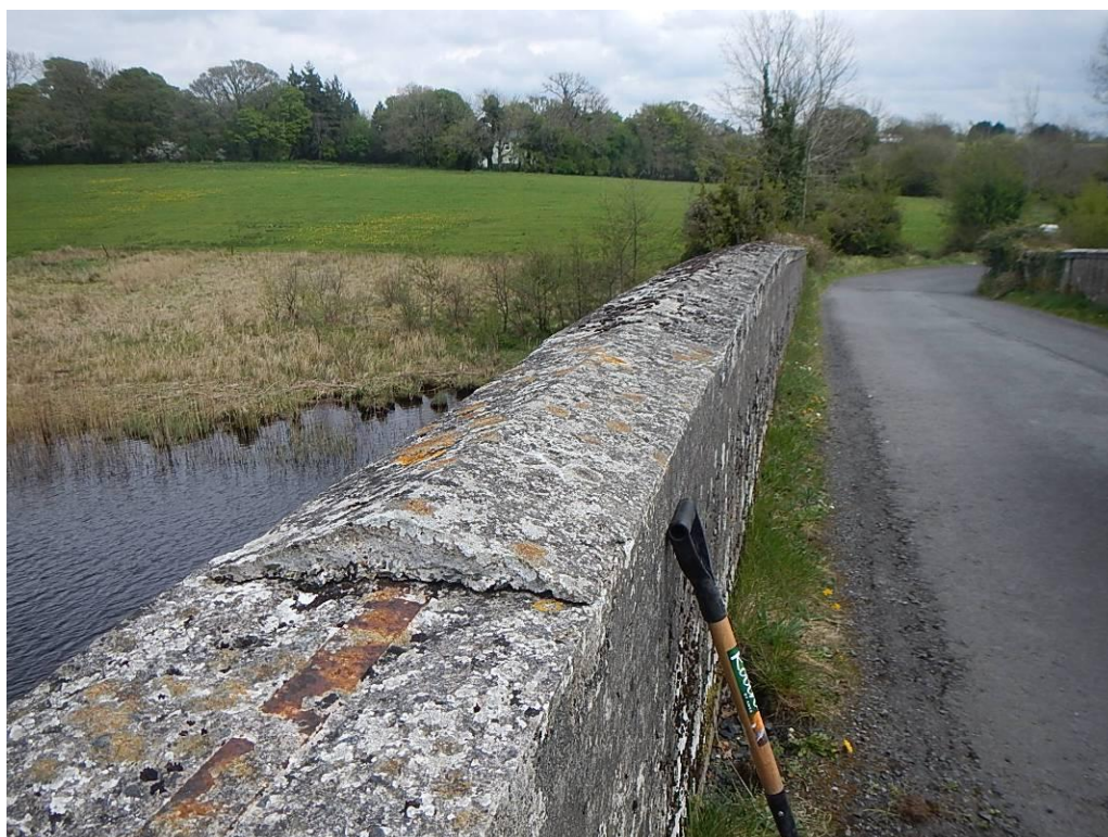
Photograph 14: Bridge Parapet / Main Longitudinal Beam (North)
