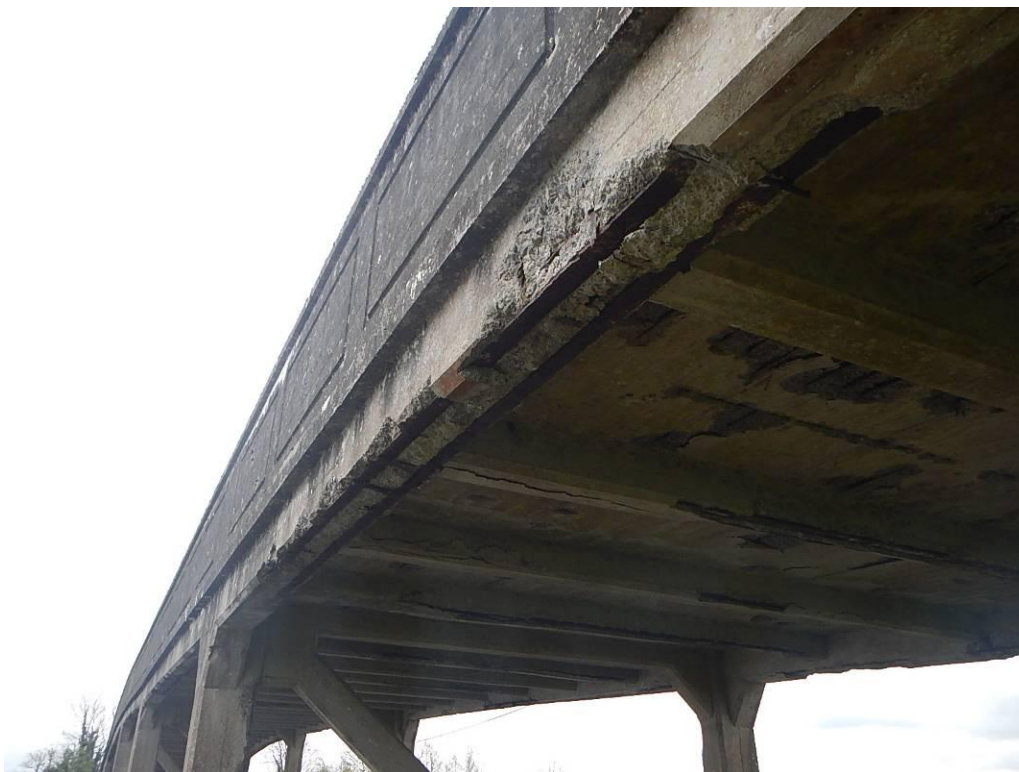
Photograph 7: Bridge Beam –Span 6
