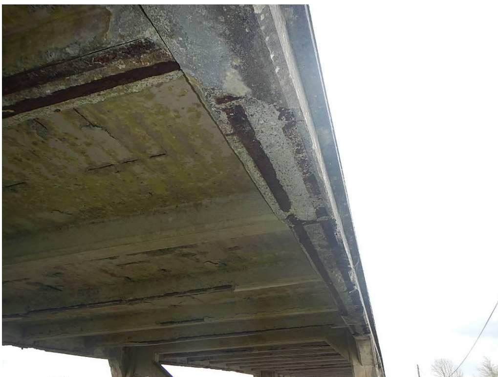
Photograph 8: Bridge Beam –Span 6
