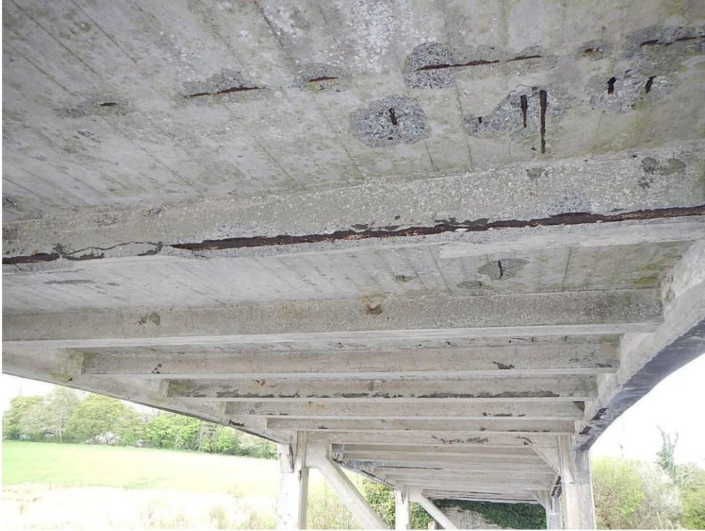
Photograph 11: Bridge Deck –Span 3
