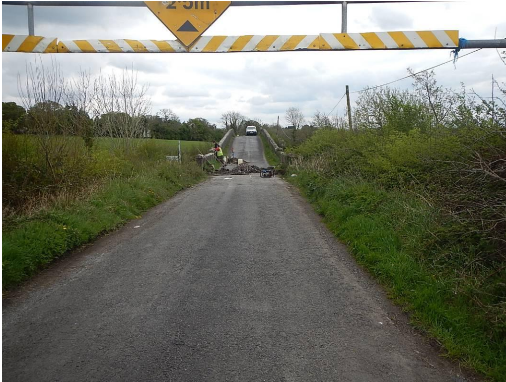
Photograph 1: Bridge Approach (west)
