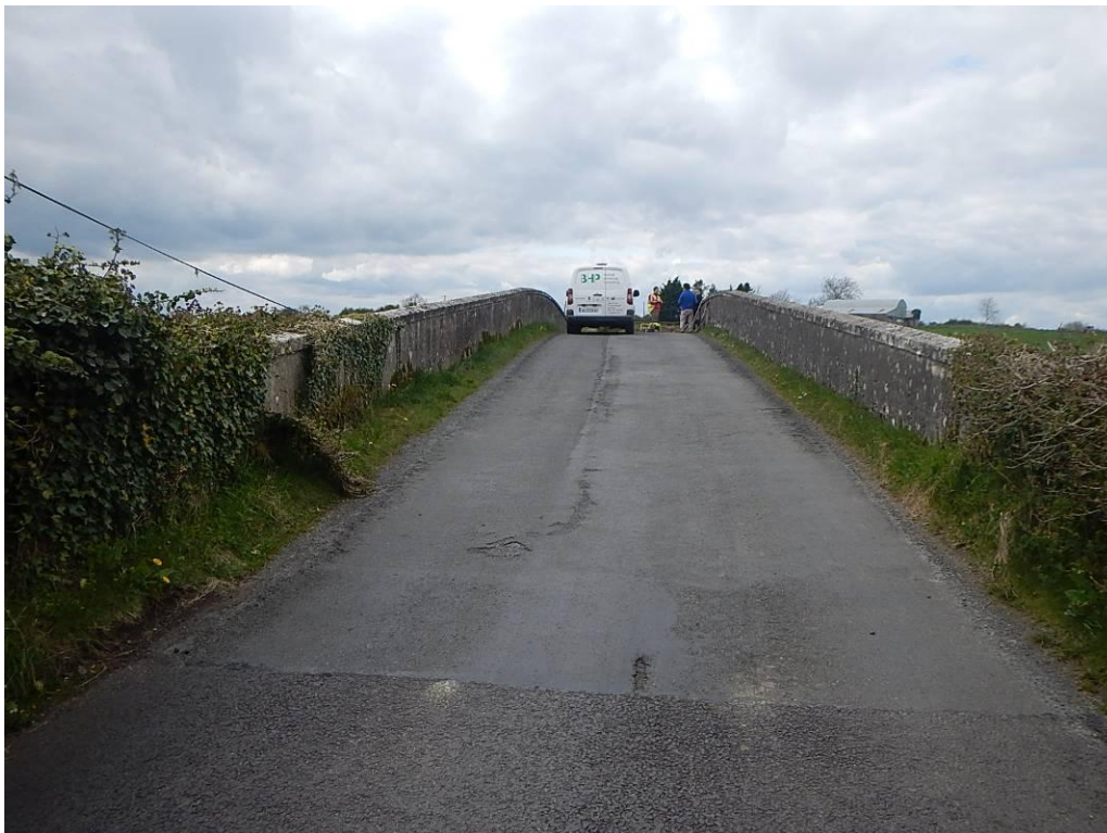
Photograph 2: Bridge Surface (East End)
