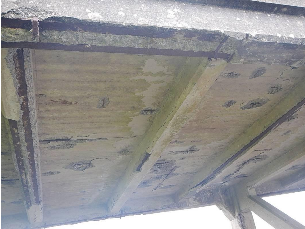
Photograph 9 Bridge Deck –Span 6
