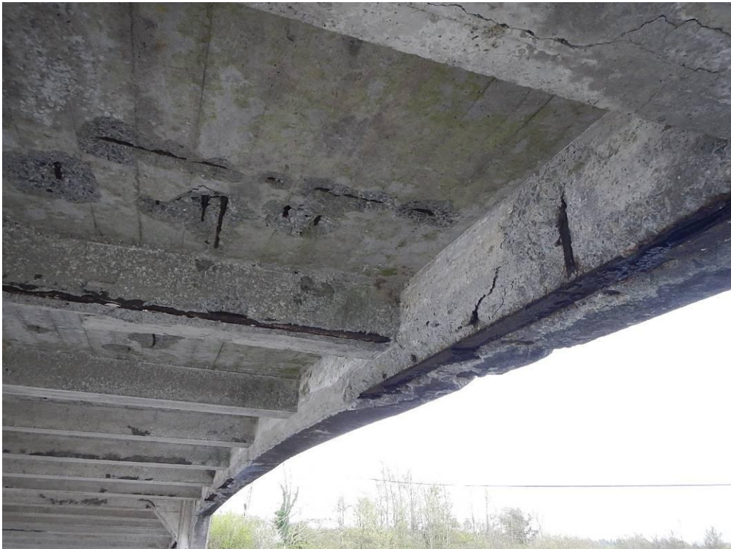
Photograph 12: Bridge Deck –Span 3
