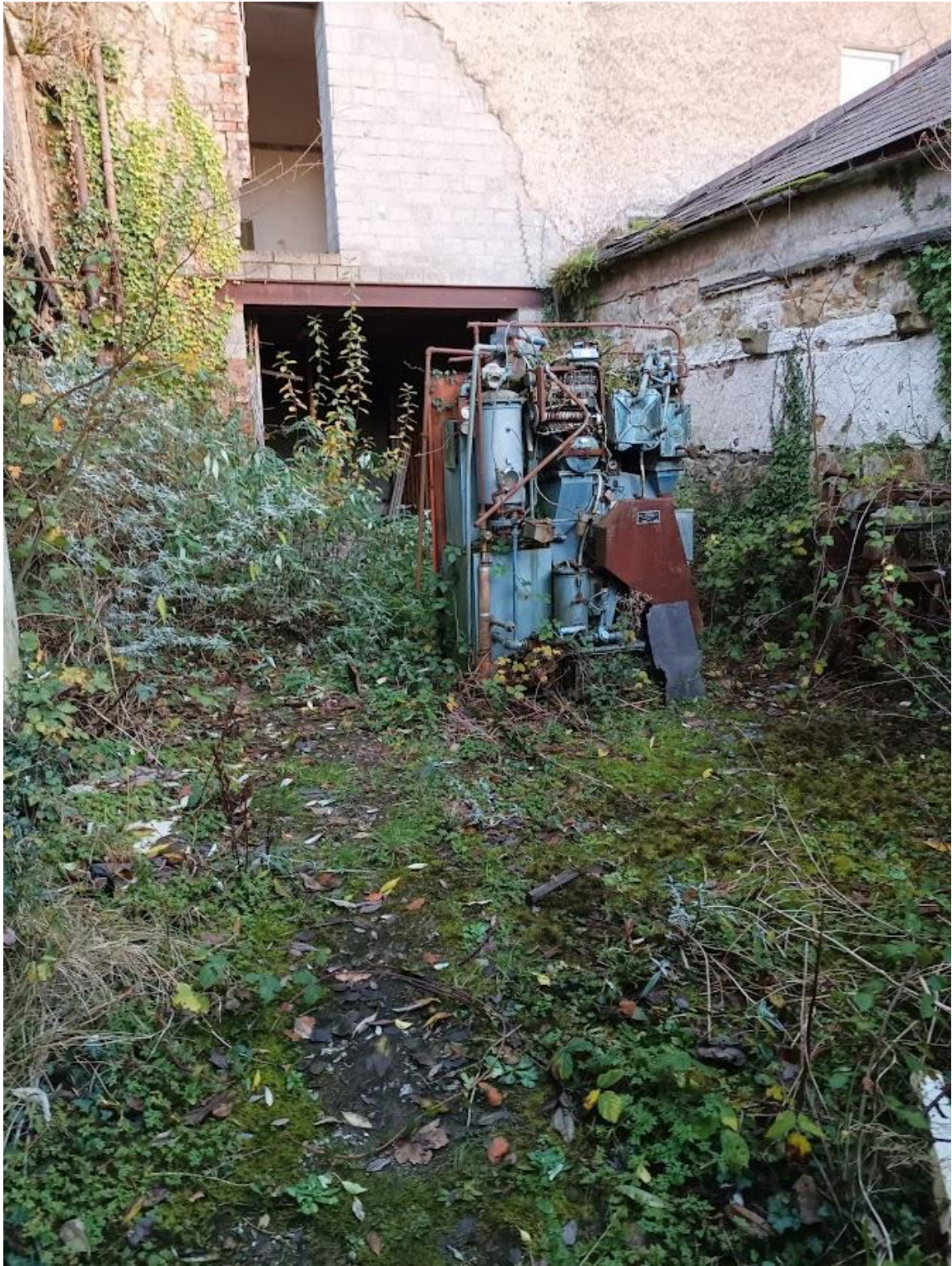
Figure 8: Rear of a derelict building accessed through double gates in laneway
