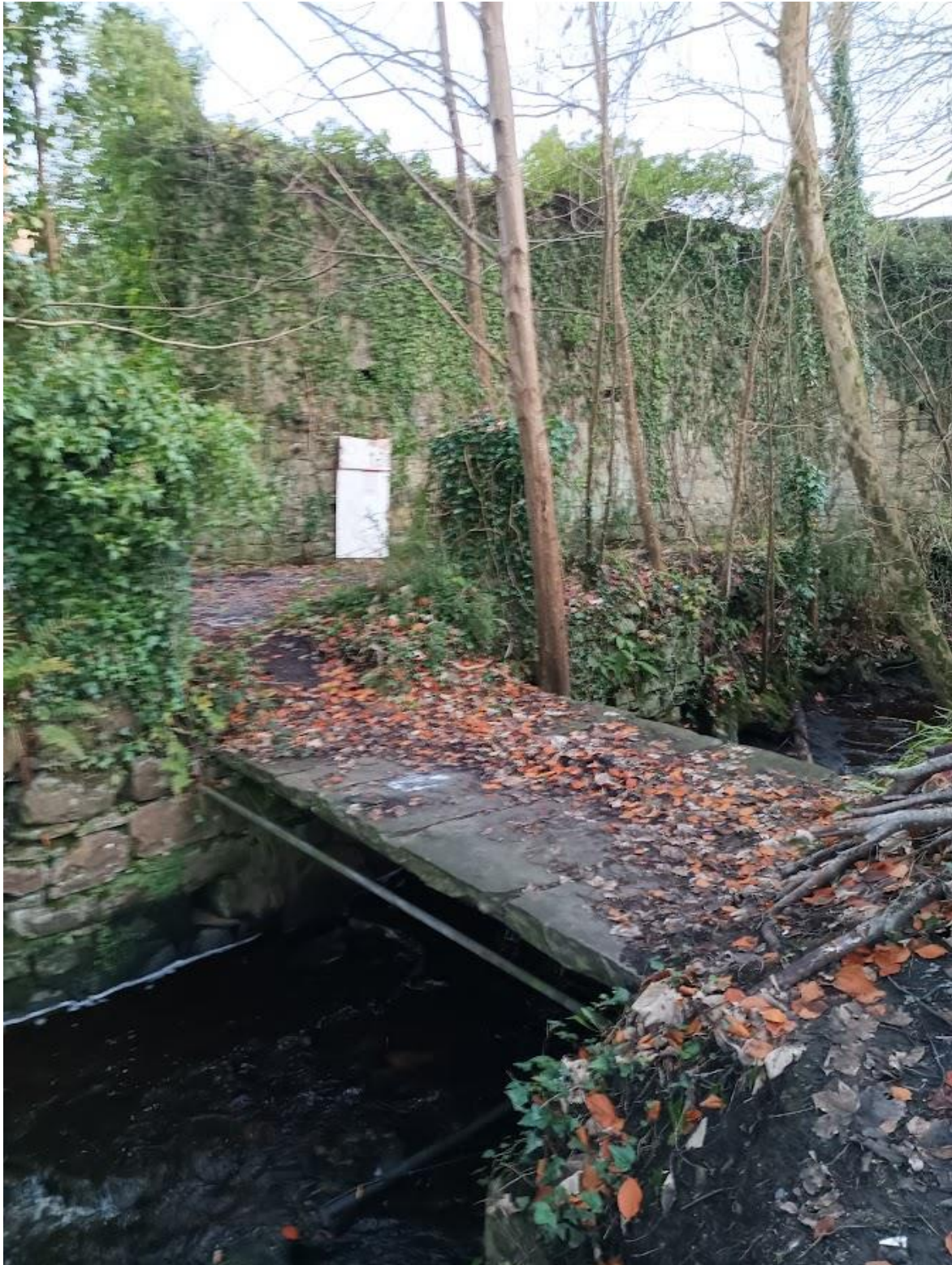
Figure 6: Old granite bridge to rear of listed buildings
