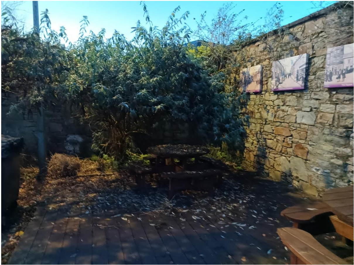
Figure 3: Corner in carpark area where Buddleia is out of control and growing up through pavement and on the old walls.
