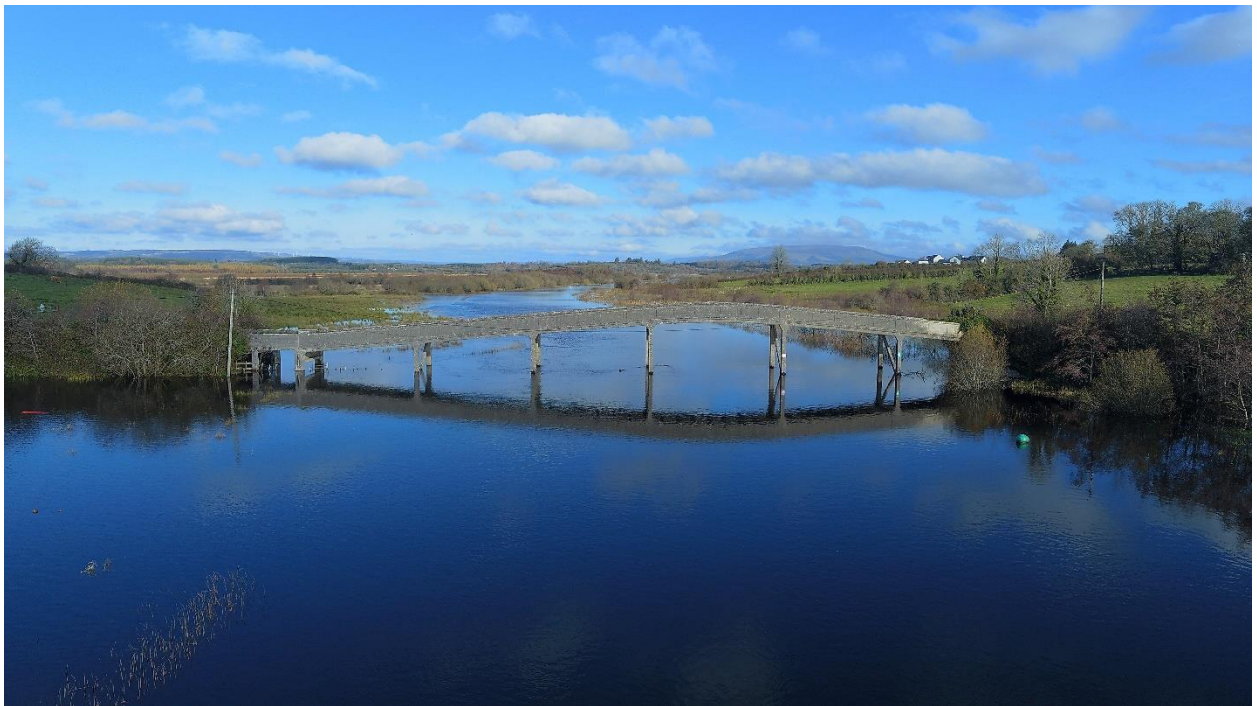
Figure 4-5: Drone footage of views around the existing Hartley Bridge (looking North towards Slieve Anierin)
