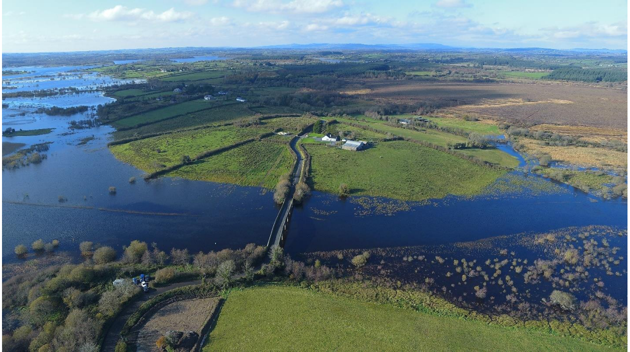
Figure 4-4: Drone footage of views around the existing Hartley Bridge (looking West)
