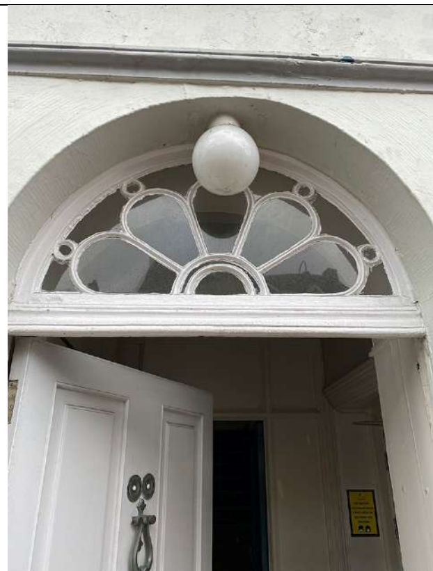
09 – Exterior view of fanlight of arched doorway
