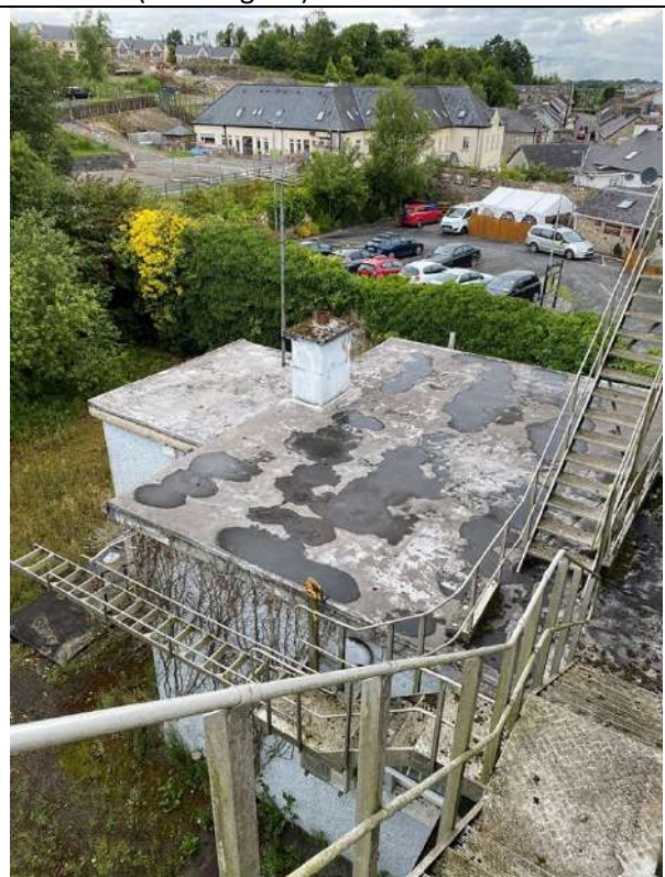
04 – Rear flat roofed extension
