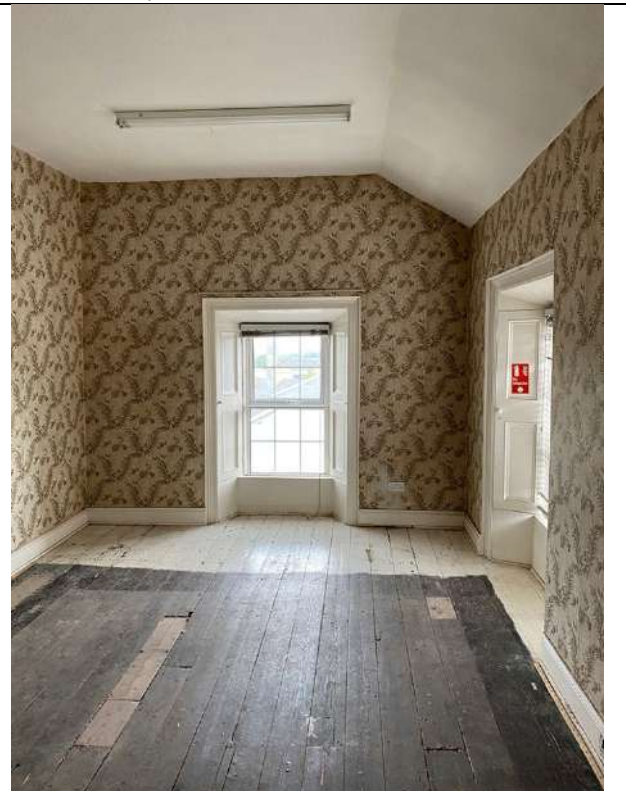
24 – 2 nd floor (former bedroom)
