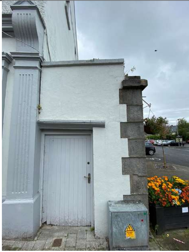
05 – existing doorway through stone wall to RHS of Bank Building
