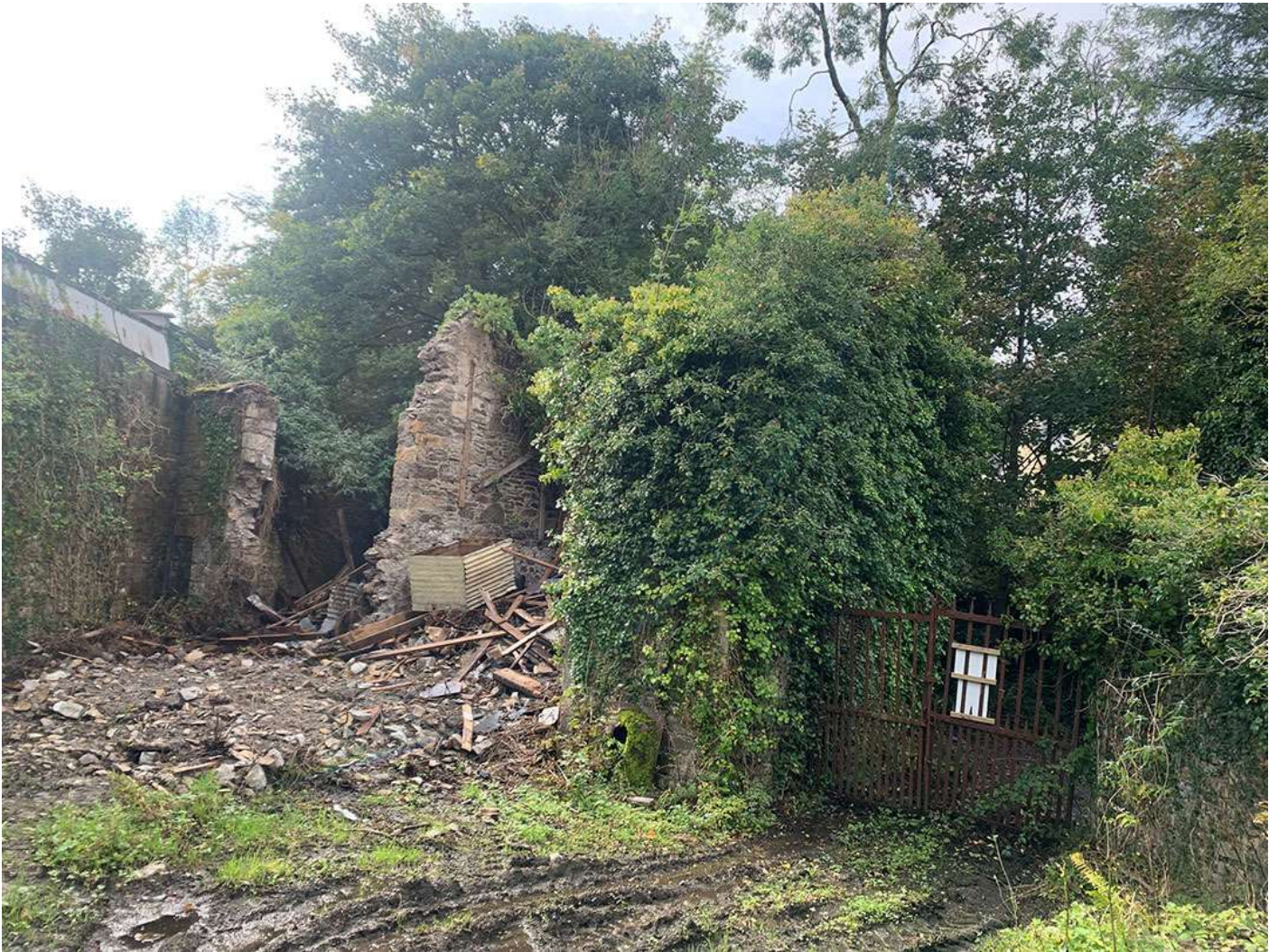
42 – External view of outbuilding #2
