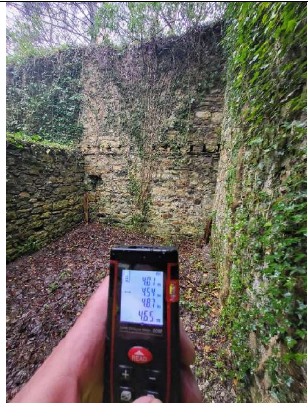
38 – Internal view of outbuilding #3
