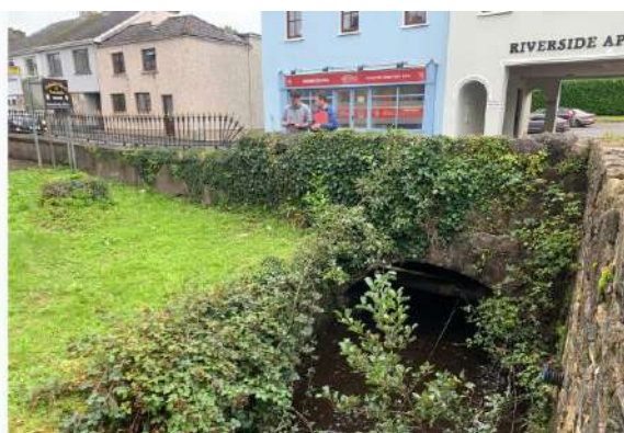
Photo 23: Carrick Road Bridge
