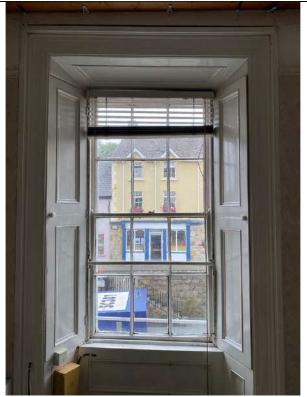
20 – Close up of window to front of building
