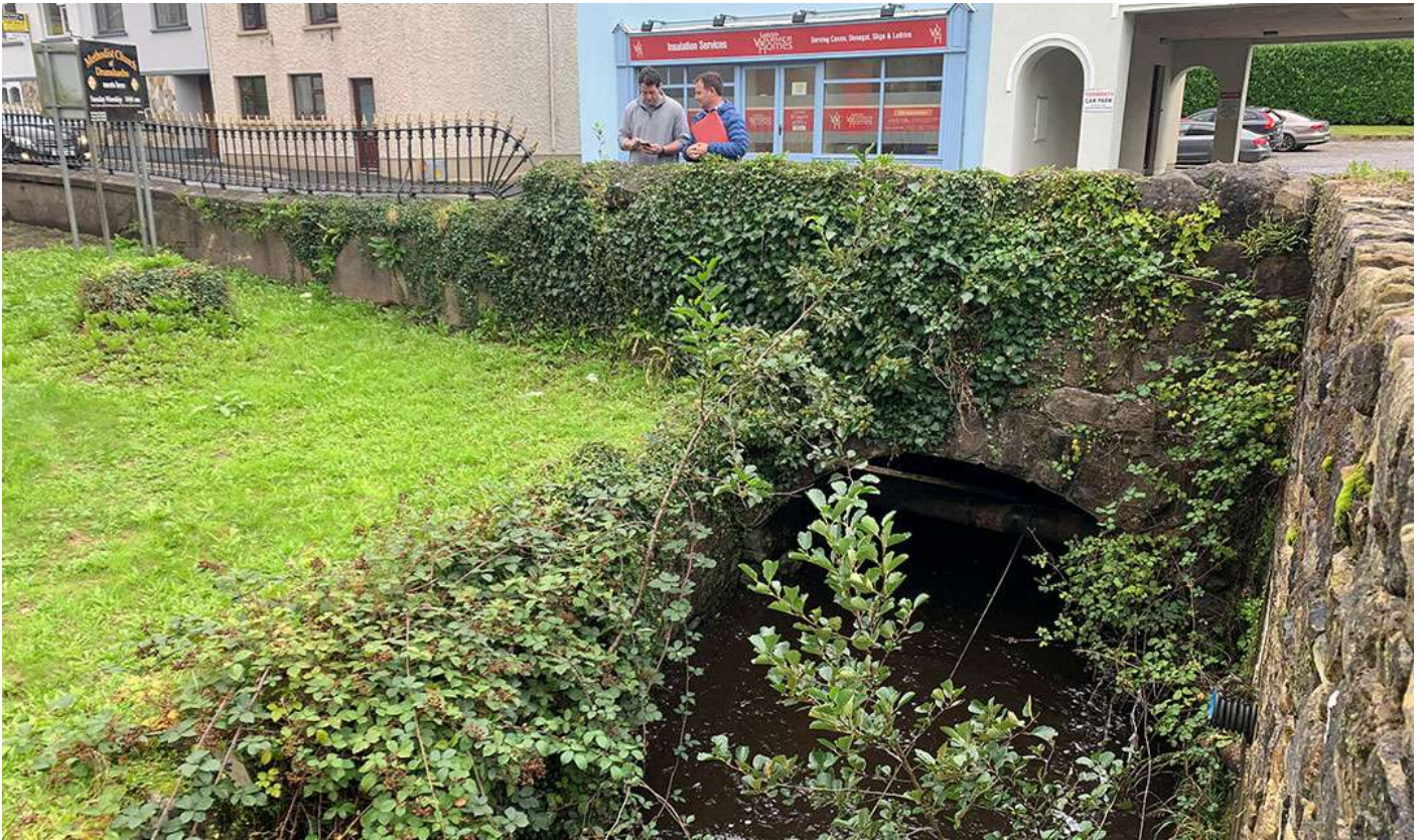
46 – View of archway of Carrick Road Bridge
