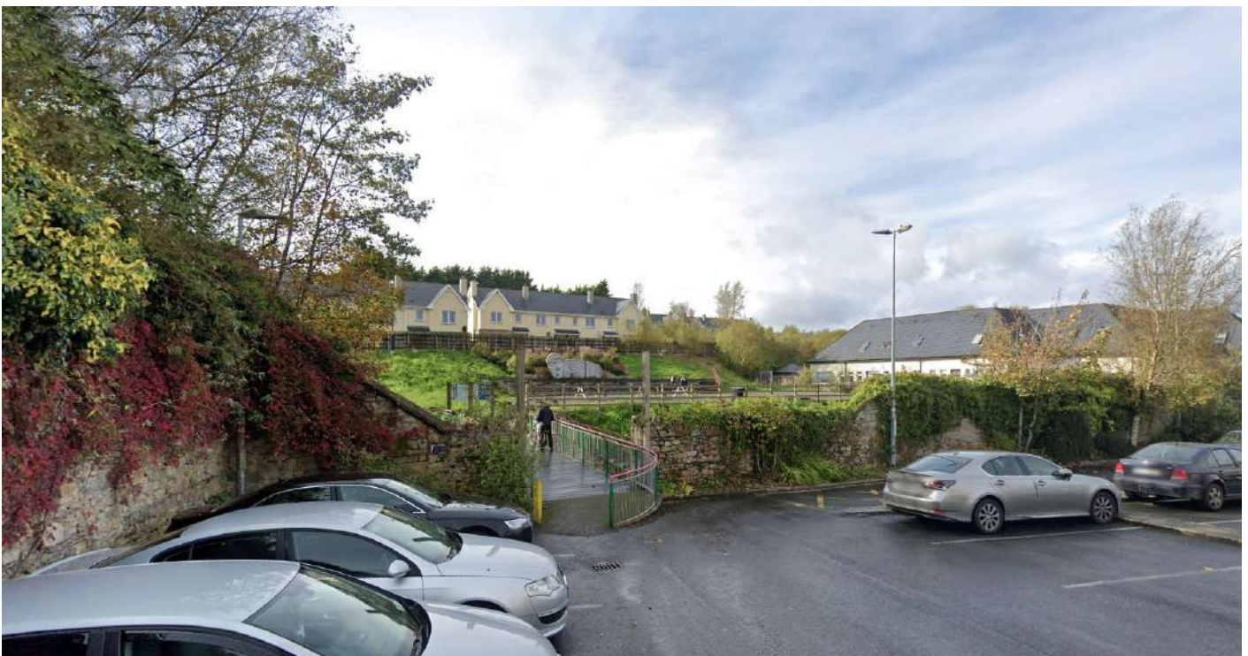
48 – Boundary wall on LHS of former bank and boundary wall to river
