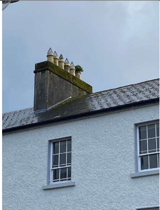
06 – Existing chimney between bank building and earley's building
