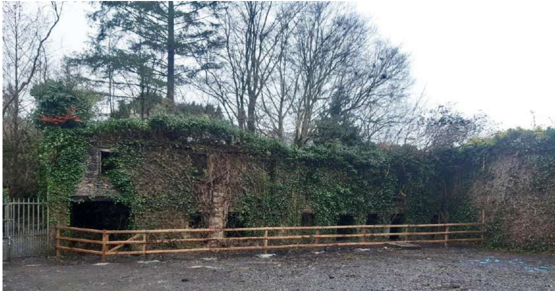
Photo 11: View of existing derelict outbuilding (building #3 – old forge)
