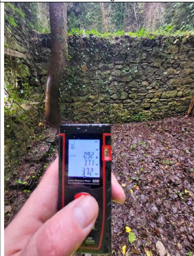
39 – Internal view of outbuilding #3
