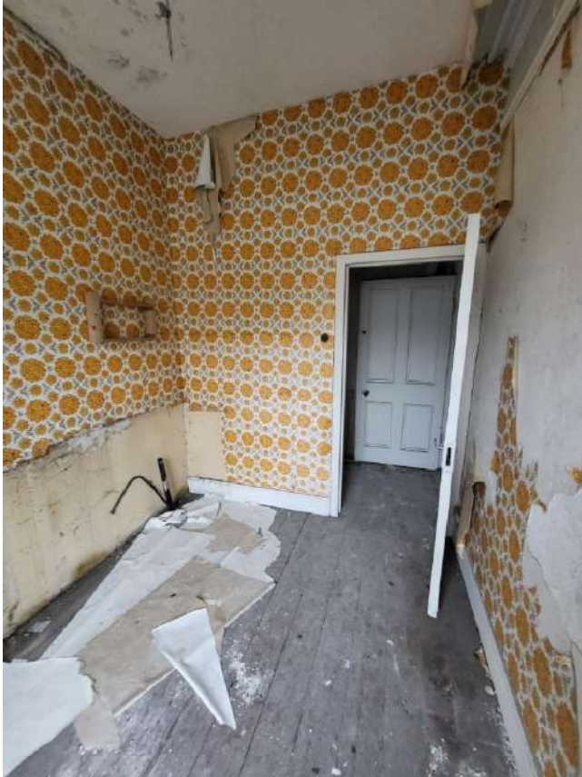
35 – rear room on 2 nd floor
