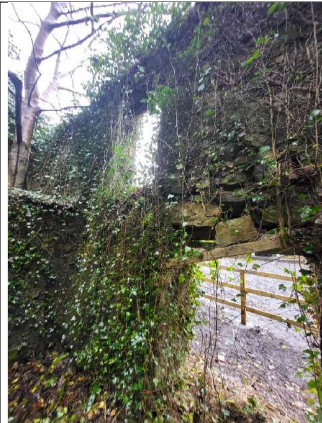
37 – Internal view of outbuilding #3
