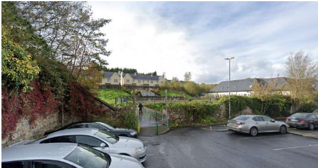
Photo 14: View of the boundary walls to car park.
