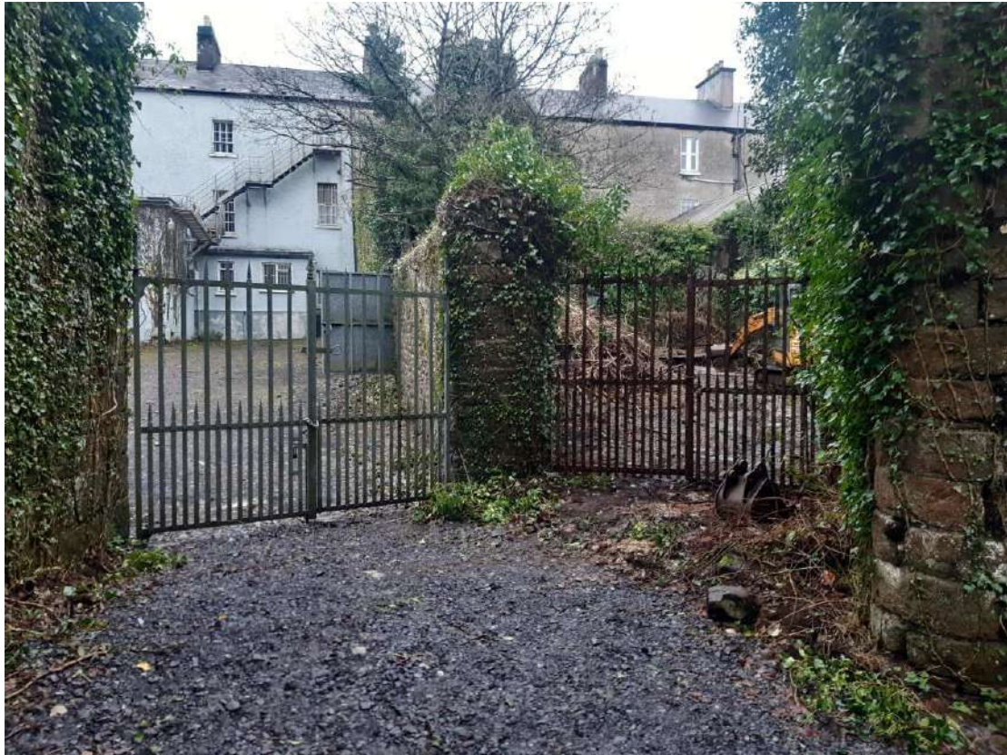
Photo 17: The current view into the rear yards of the former Bank of Ireland (LHS) and Earley' (RHS)
