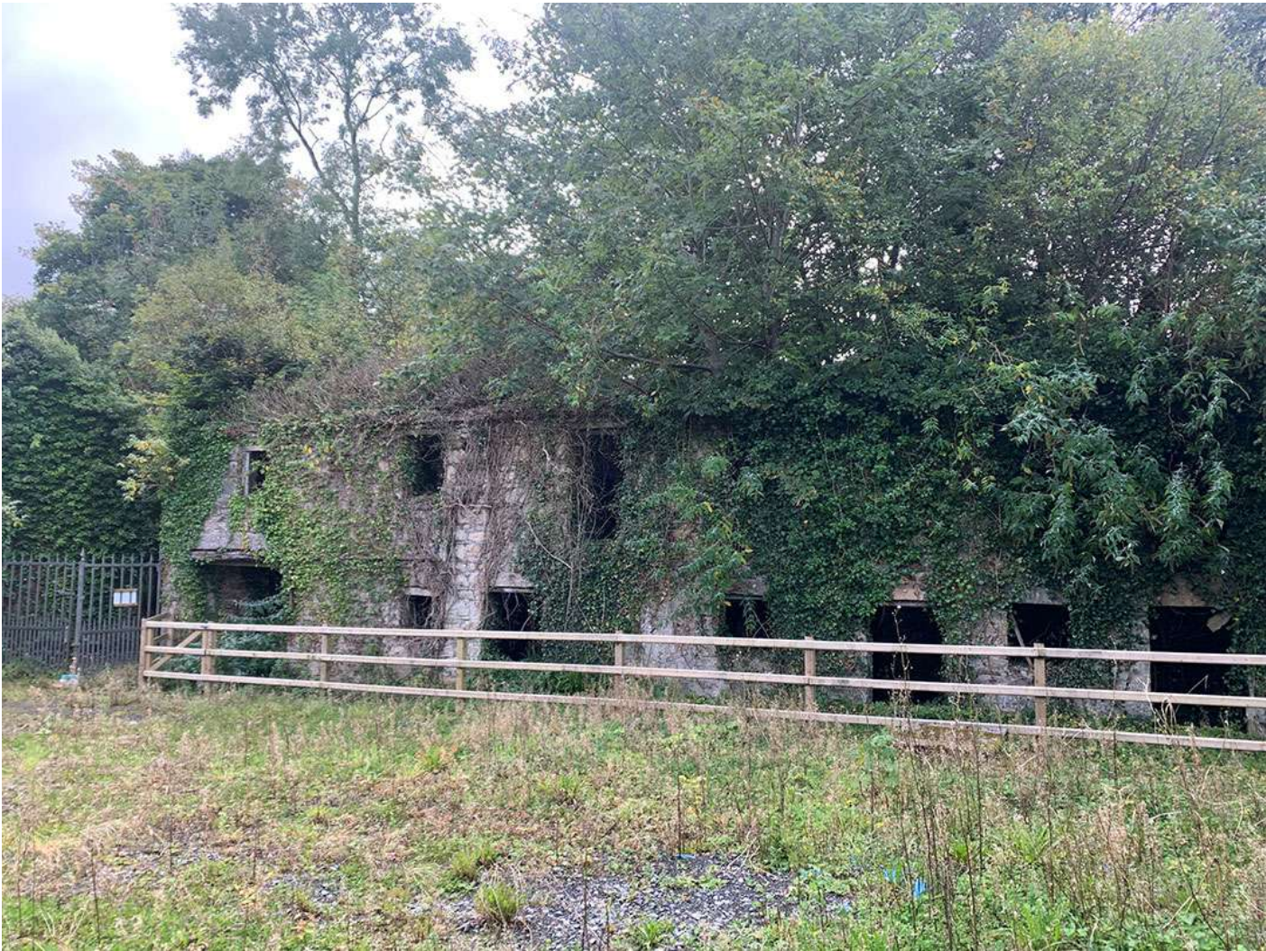
41 – External view of outbuilding #3 (old forge)
