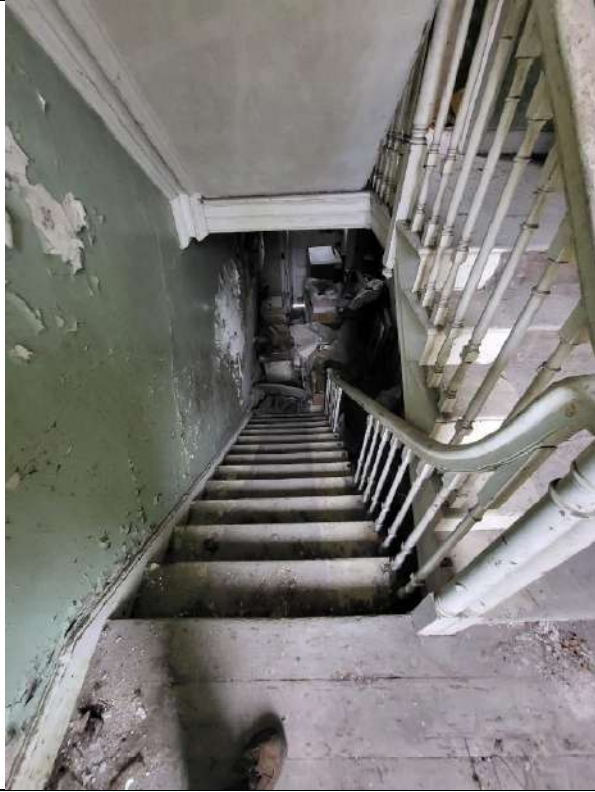
29 – Staircase (view from landing level)
