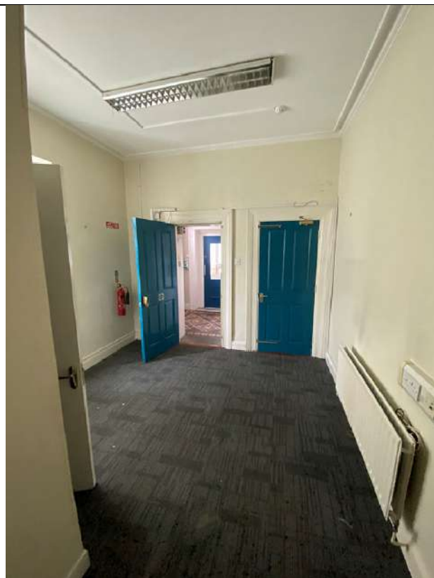
10 – front room to left of hallway
