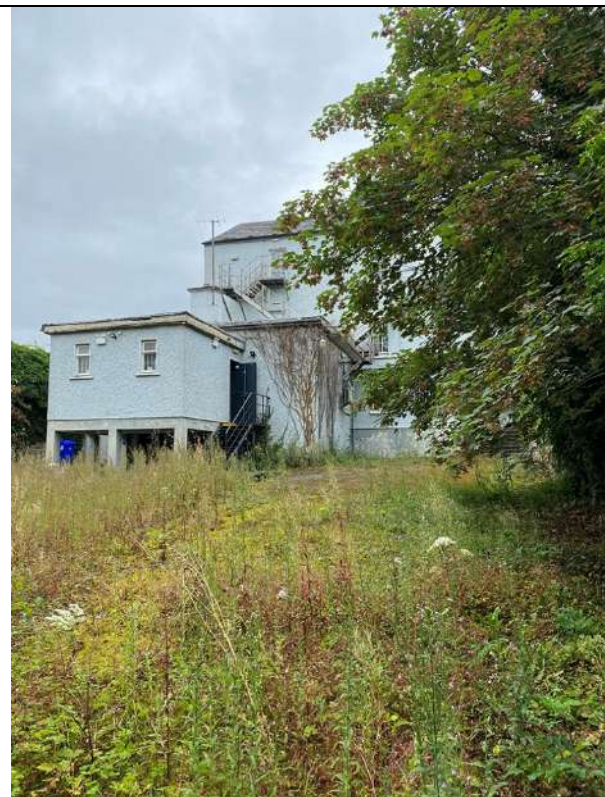
03 – Rear non-original extension and existing yard
