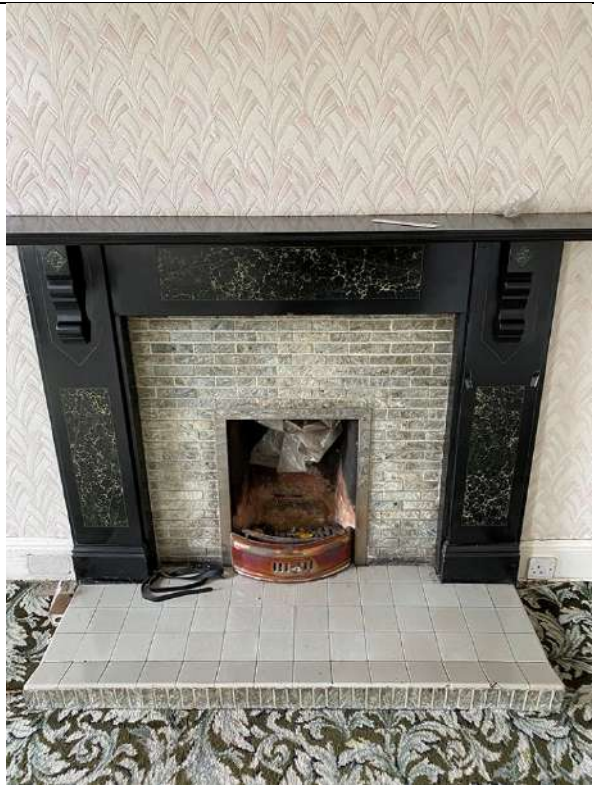
19 – Fireplace on first floor
