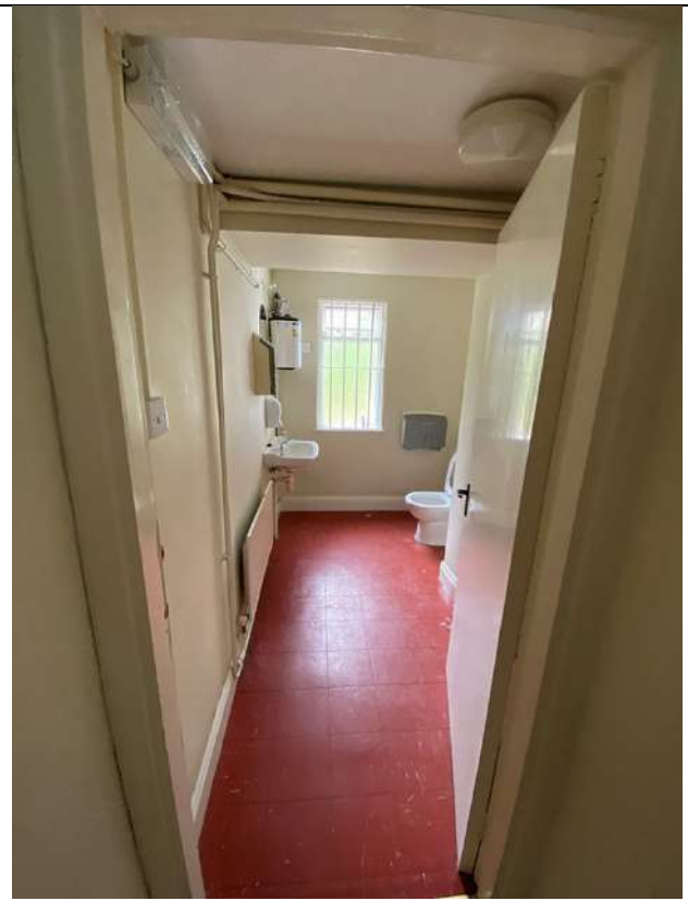
16 – View to WC extension to rear (off hallway)
