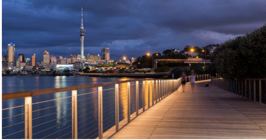
Guardrail with lighting - Installed under the handrail
