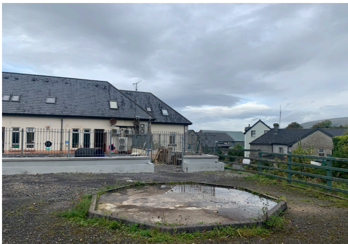
Remove brick edge, change timber fence to guardrail (Black) • Match the new boundary treatment
