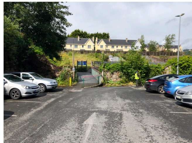
Lower the stone wall and add swale to the front • permit view to People's park
