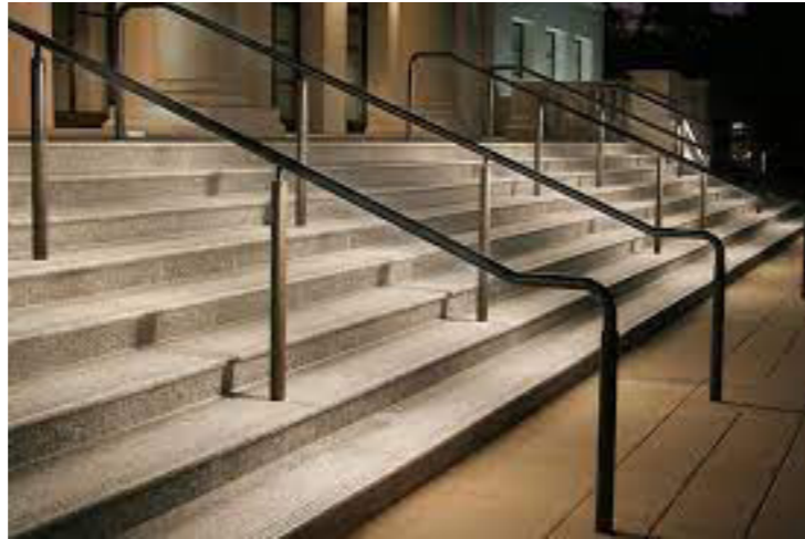
Stepped access with lighting - Installed to recess in handrail
