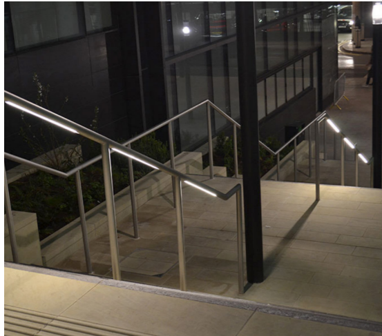
Stepped access with lighting - Installed to recess in handrail
