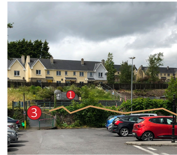
Wall & overgrown areas - limiting visual connections
