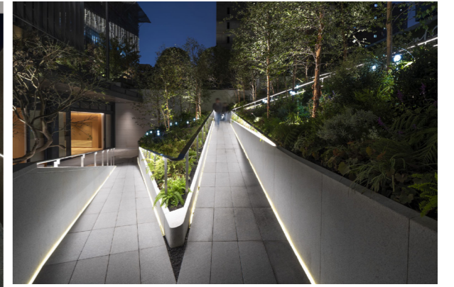
Ramped access with lighting - Along the surface edge
