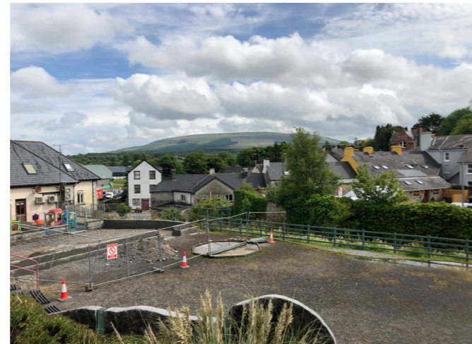
Wider landscape views after replacing the timber fence to guardrail
