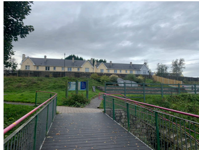
Paint existing pink railing to black • Match the new boundary treatment
