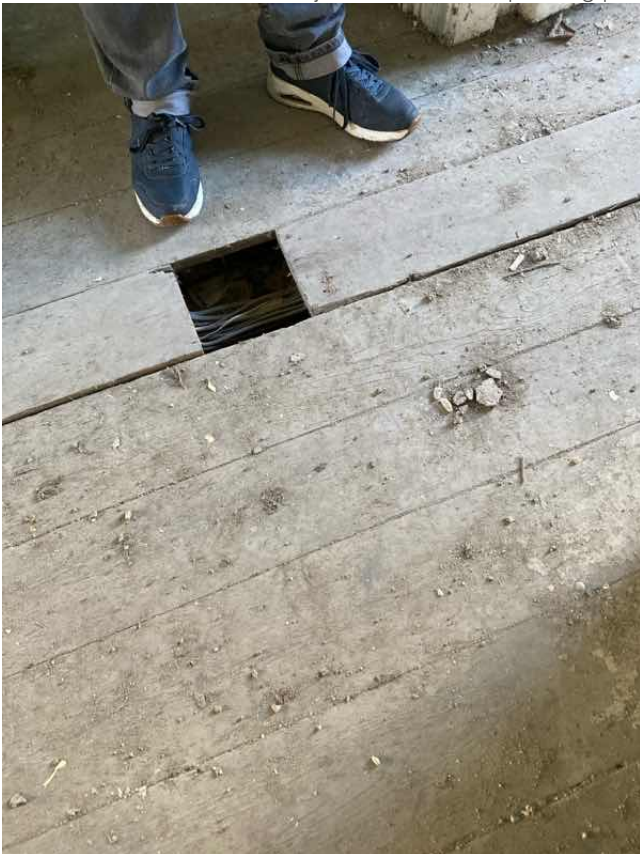
Floor boards indicate that all joist on first floor spanning parallel to front wall of building.
