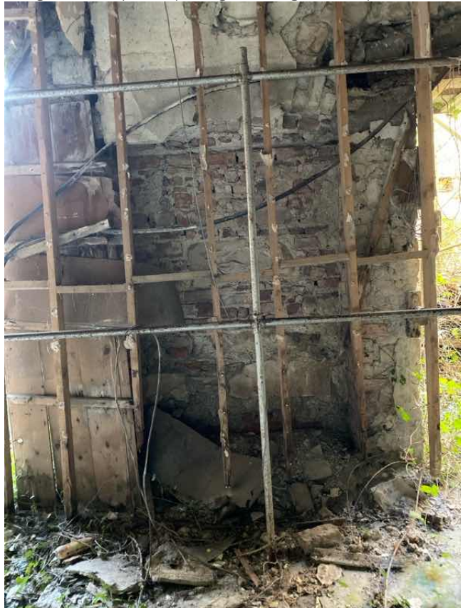
81 Middle masonry pier on back wall has opening in middle of same (most likely an original window that has been bricked up). This weakens the load bearing pier, so we would be recommending to build up the opening to strengthen the pier.
