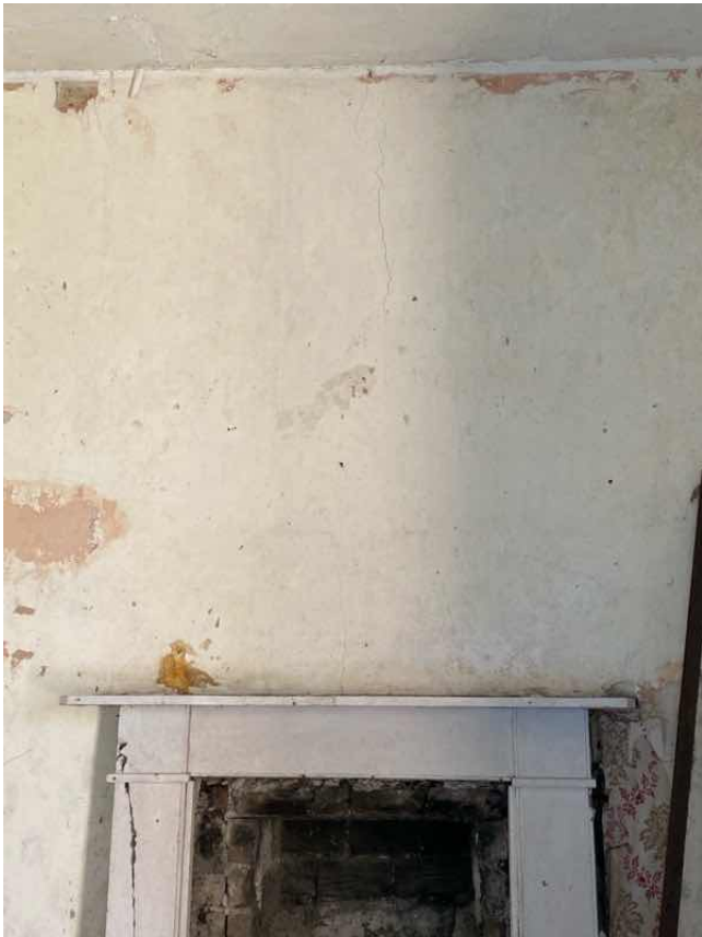
Evidence of cracking in wall above fire place. Masonry partially collapsed in fire place
