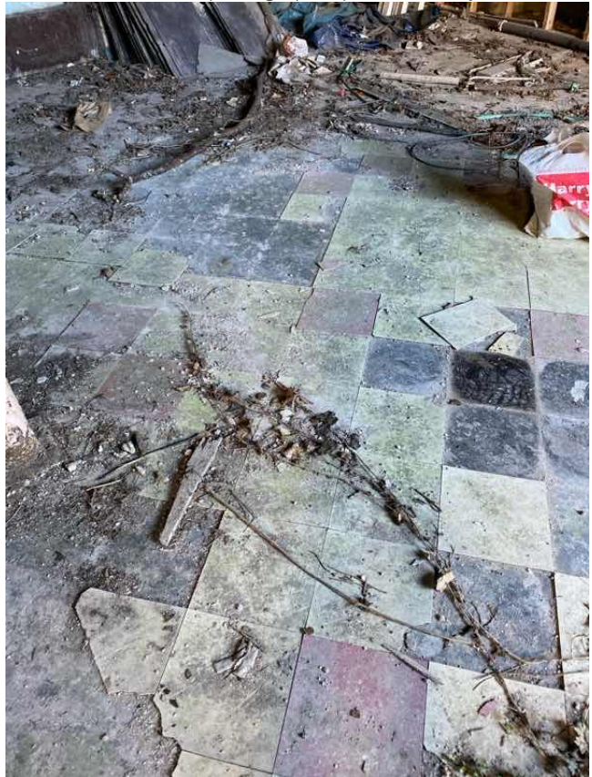
82 Concrete floor slab in place. Unclear if DPM and insulation exist under the same. Opening up required to verify this.
