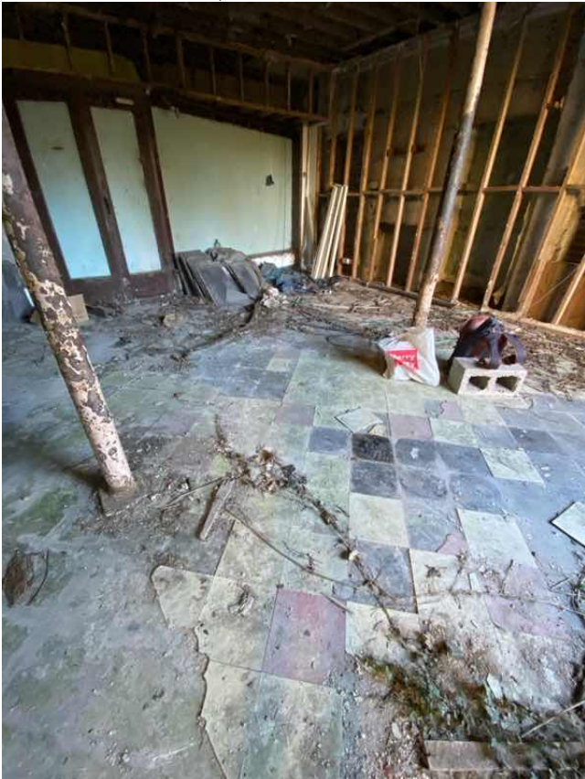
82 Concrete floor slab in place. Unclear if DPM and insulation exist under the same. Opening up required to verify this.
