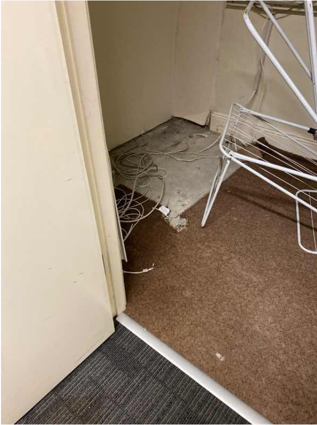
Carpeted floor on ground bearing concrete slab
