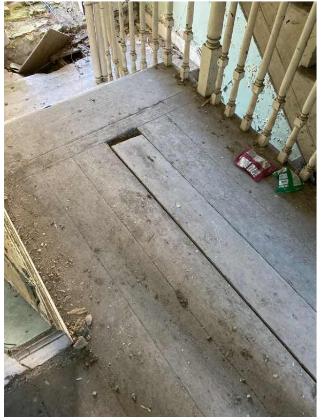
Floor boards indicate that all joist on first floor spanning parallel to front wall of building.
