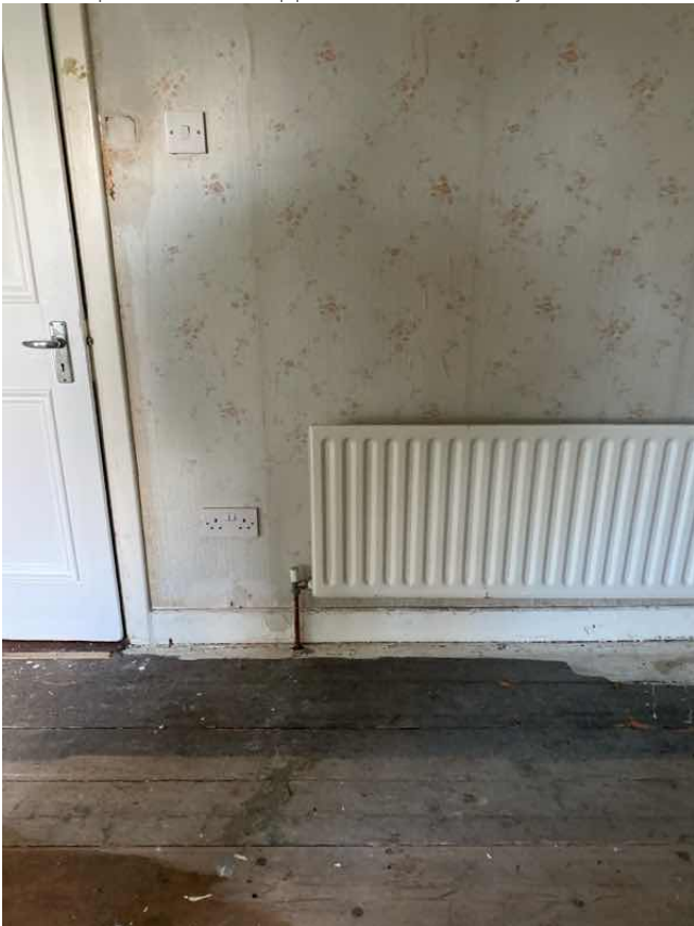
Internal partition wall supported off the floor joist
