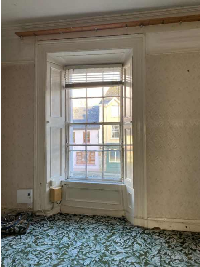
Timber linings around existing sash windows
