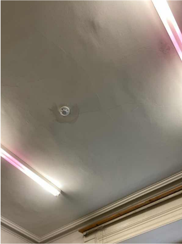
Cieling in satisfactory condition, observed hairline cracks at the lights
