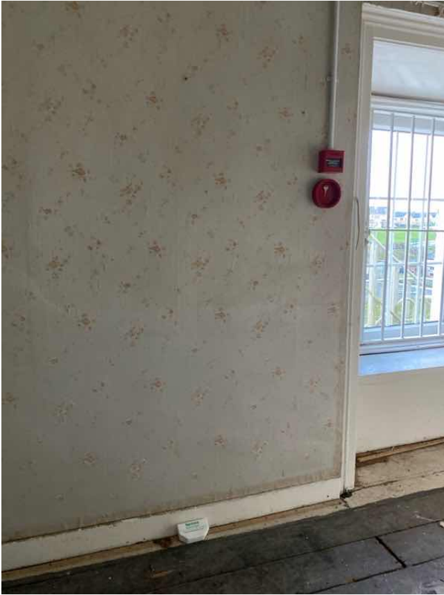
Rear wall drylined
