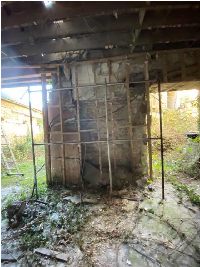
81 Middle masonry pier on back wall has opening in middle of same (most likely an original window that has been bricked up). This weakens the load bearing pier, so we would be recommending to build up the opening to strengthen the pier.
