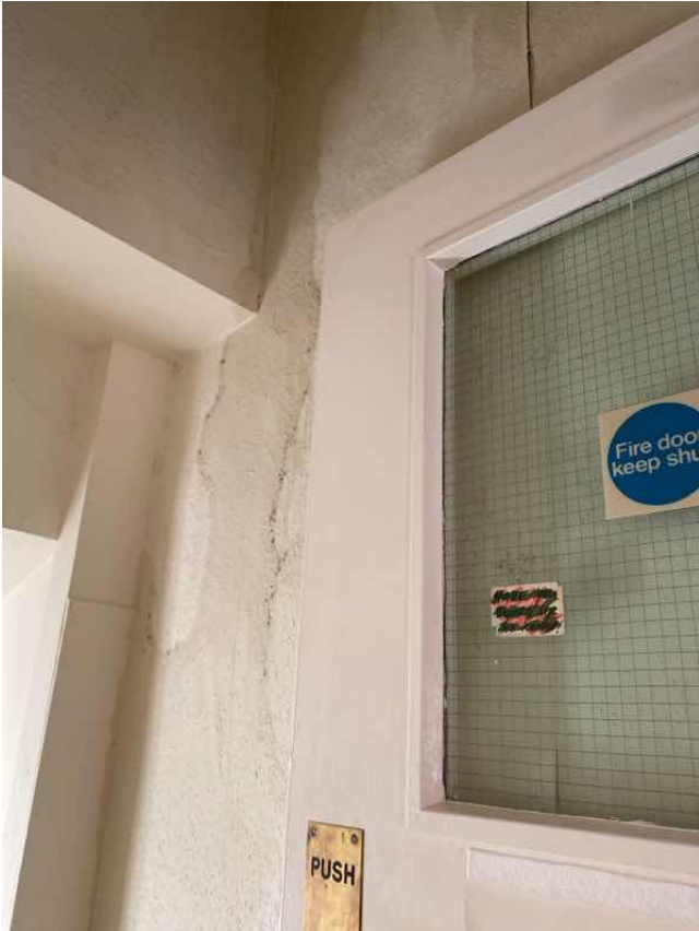
Significant ingress of water on rear external wall, wall damp to touch indicates an active leak
