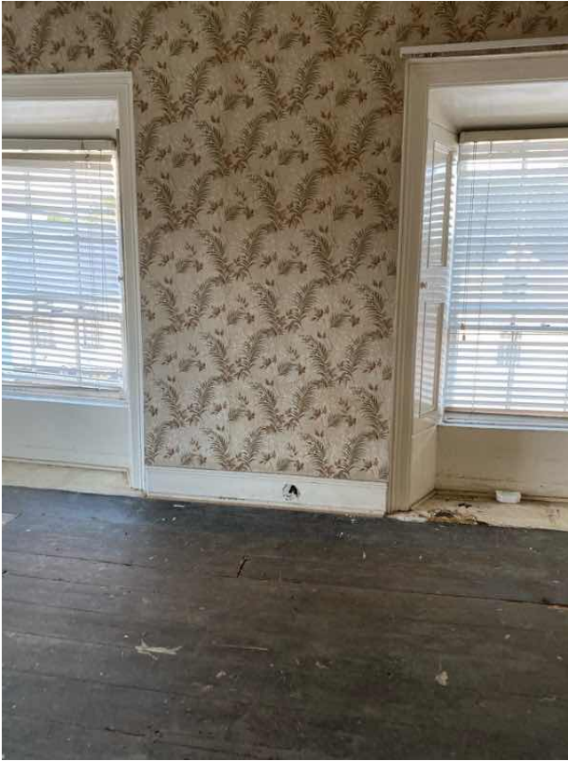
All external walls dry lined
