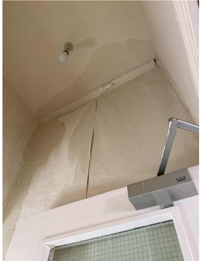
Significant ingress of water on rear external wall, wall damp to touch indicates an active leak
