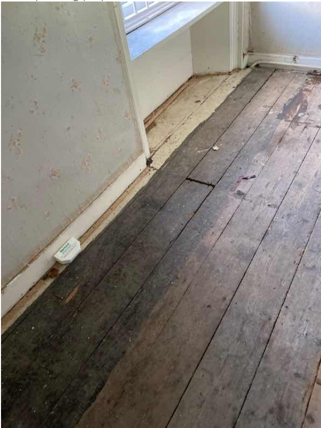
Joist spanning perpendicular to the rear exterior wall.
