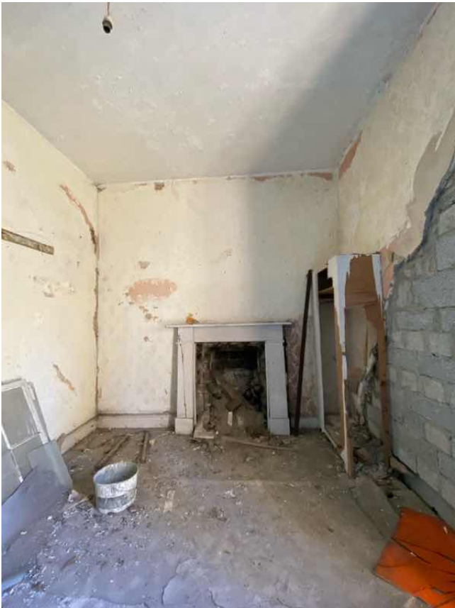
Evidence of cracking in wall above fire place. Masonry partially collapsed in fire place
