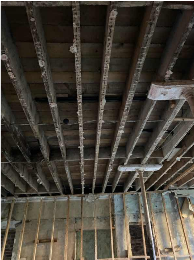
Floor Joist are 250x50 @ 300 centres.
