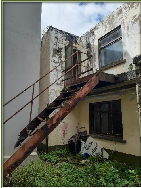
Plate 1 – Building at the Back of the Site
