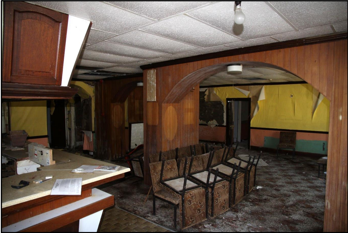
Plate 6: The ground floor of the northern post-1908 extension looking through the archway which carries the old gable of the pre-1908 building
