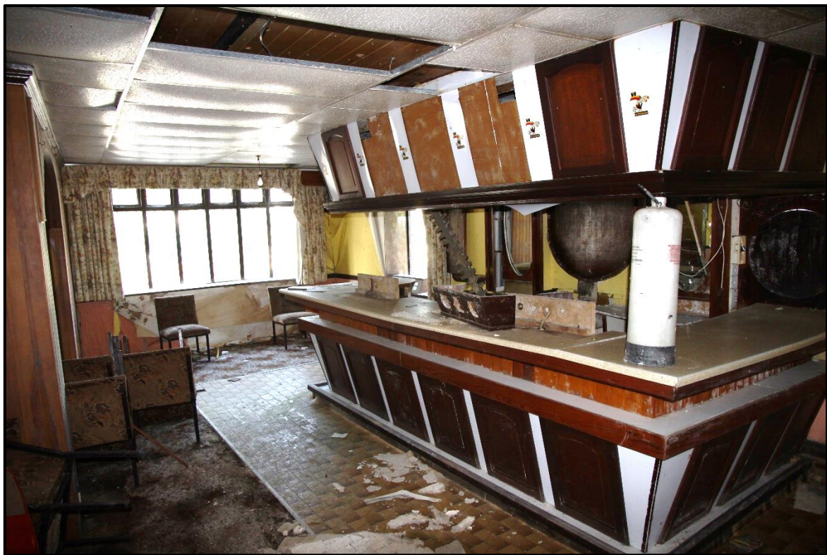
Plate 5: The ground floor of the northern post-1908 extension
