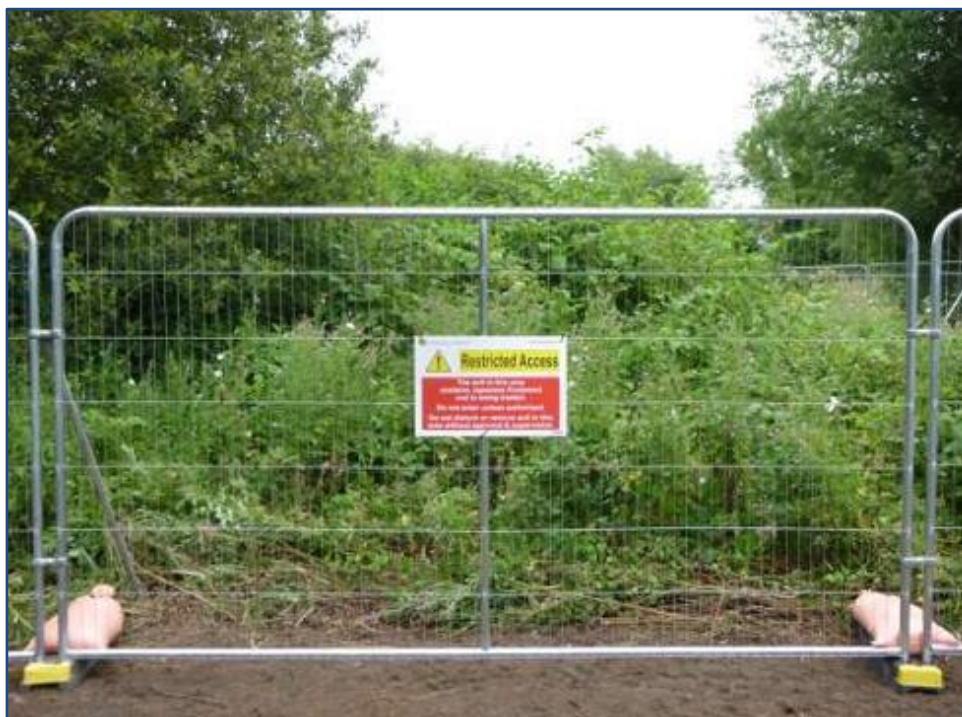
Plate 4-1: Heavy Duty Heras Fencing
