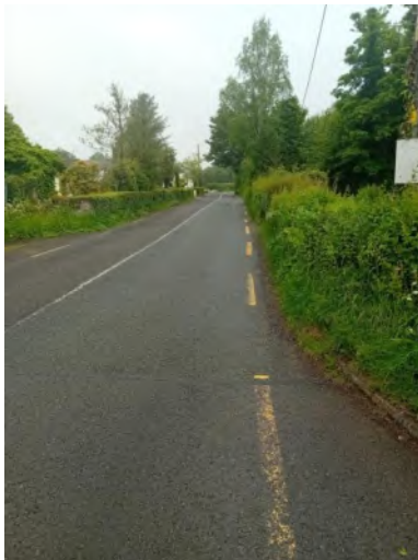
Plate 1. Looking north from junction with R281 along the R282, route for sewer pipe.
