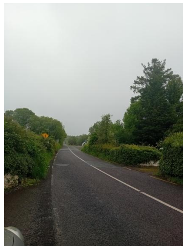
Plate 2. Looking north along R282 towards Gublaun Estate.
