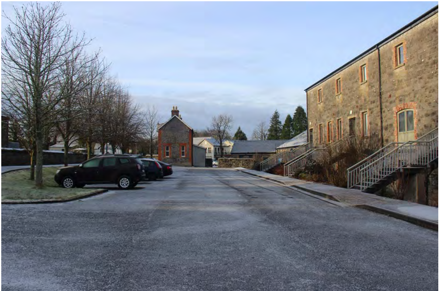
J991_P38 View of Eastern Elevation of Former Station Masters House
