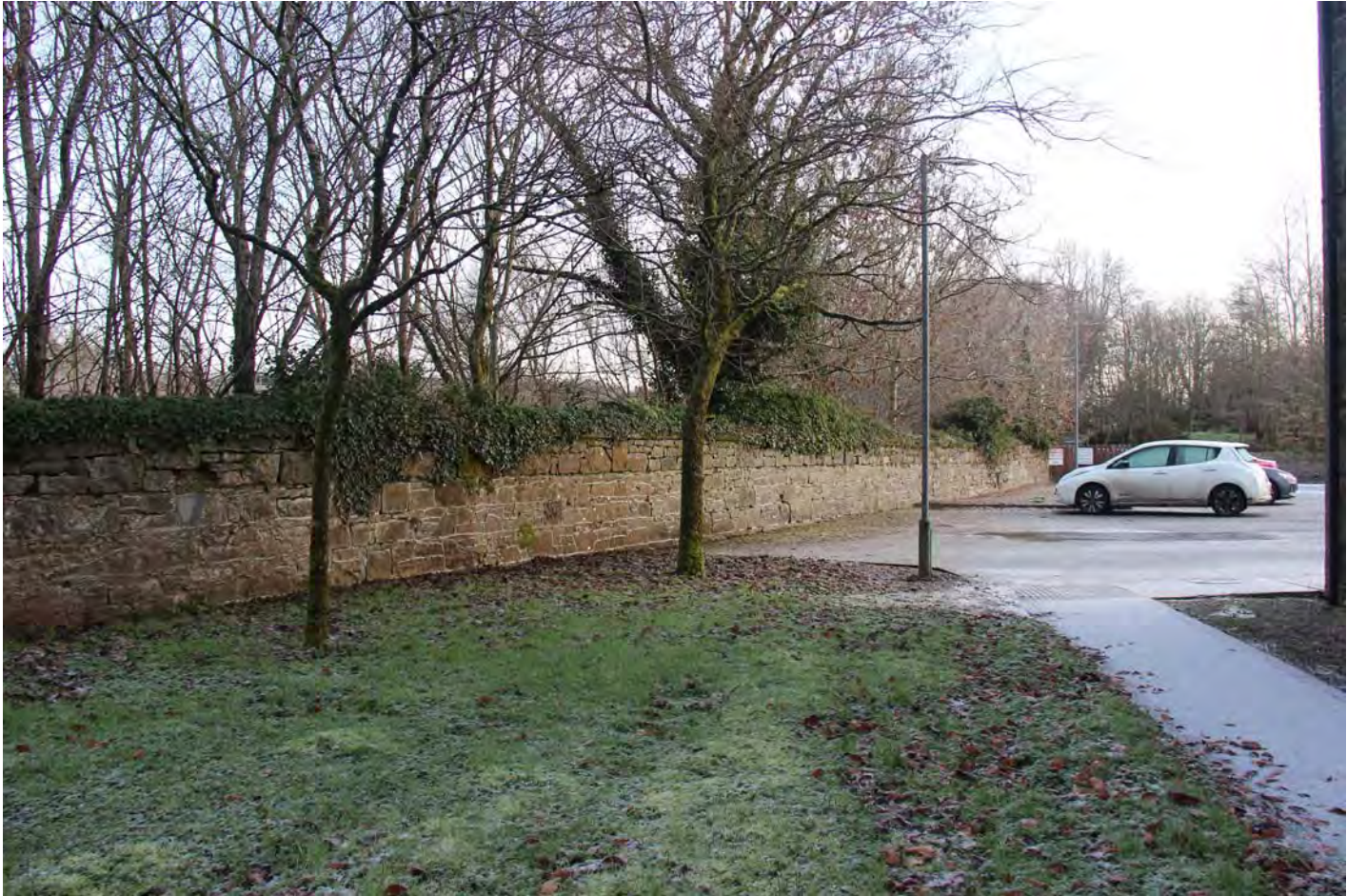
J991_P12 Existing Boundary Wall Section B
