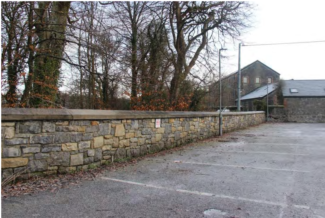
Photograph 17 - Section E Modern Stone-faced wall with Concrete Cap
