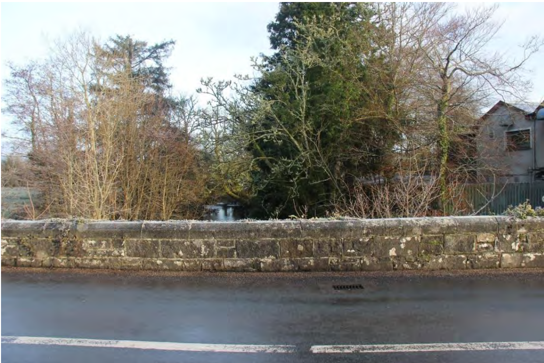
Photograph 20 - Stone Bridge over tributary with cut stone capping.
