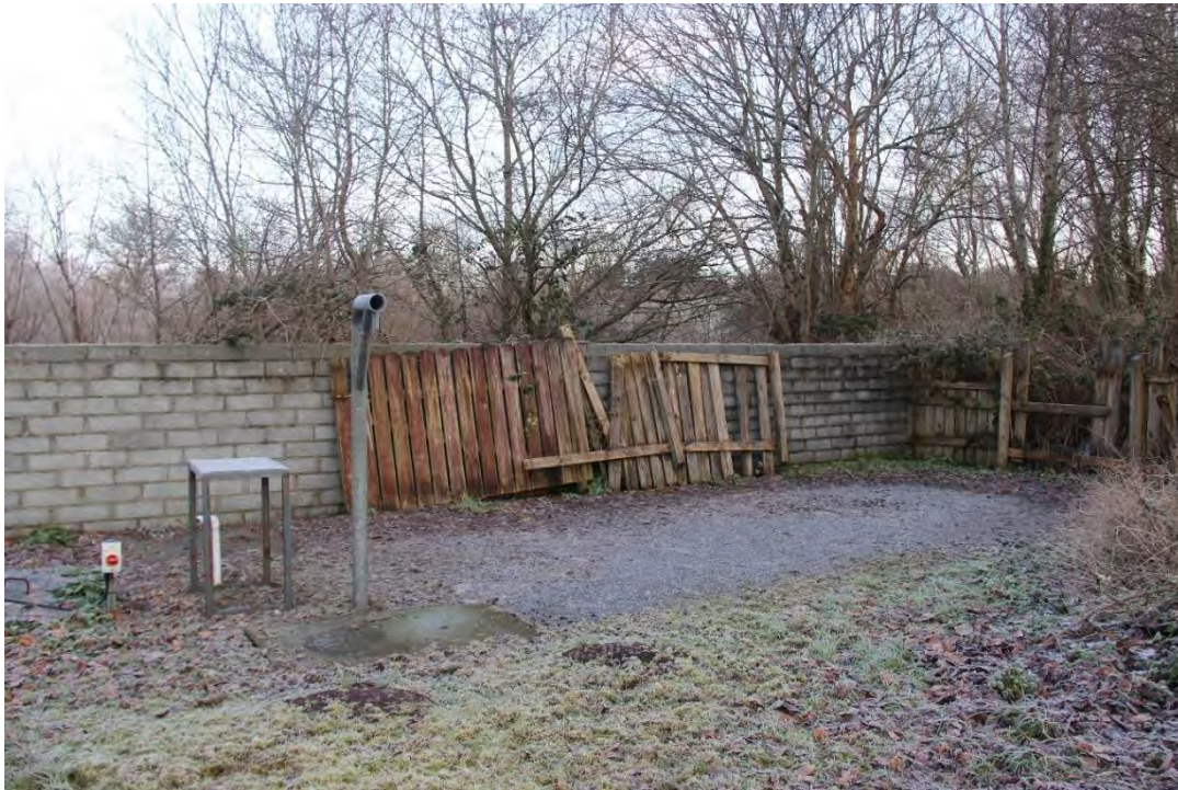
Photograph 7 - Section A Existing Boundary Wall
