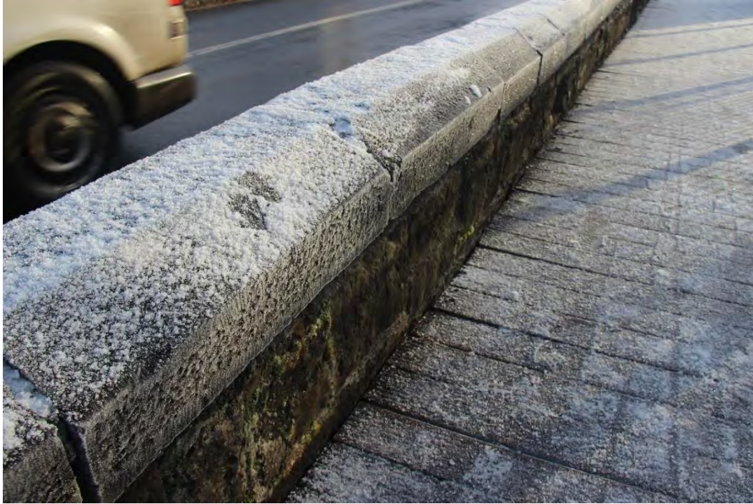
Photograph 21 - Detail of Cut Stone Capping
