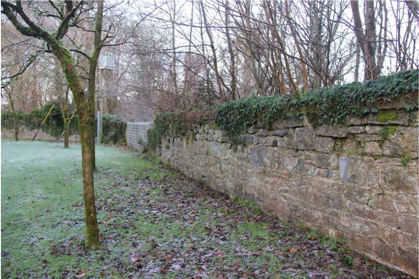
J991_P10 Existing Boundary Wall Section B to Section C
