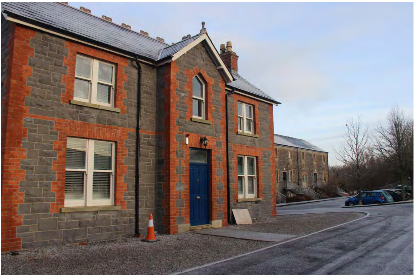
J991_P30 View of Southern Elevation of Former Station Masters House
