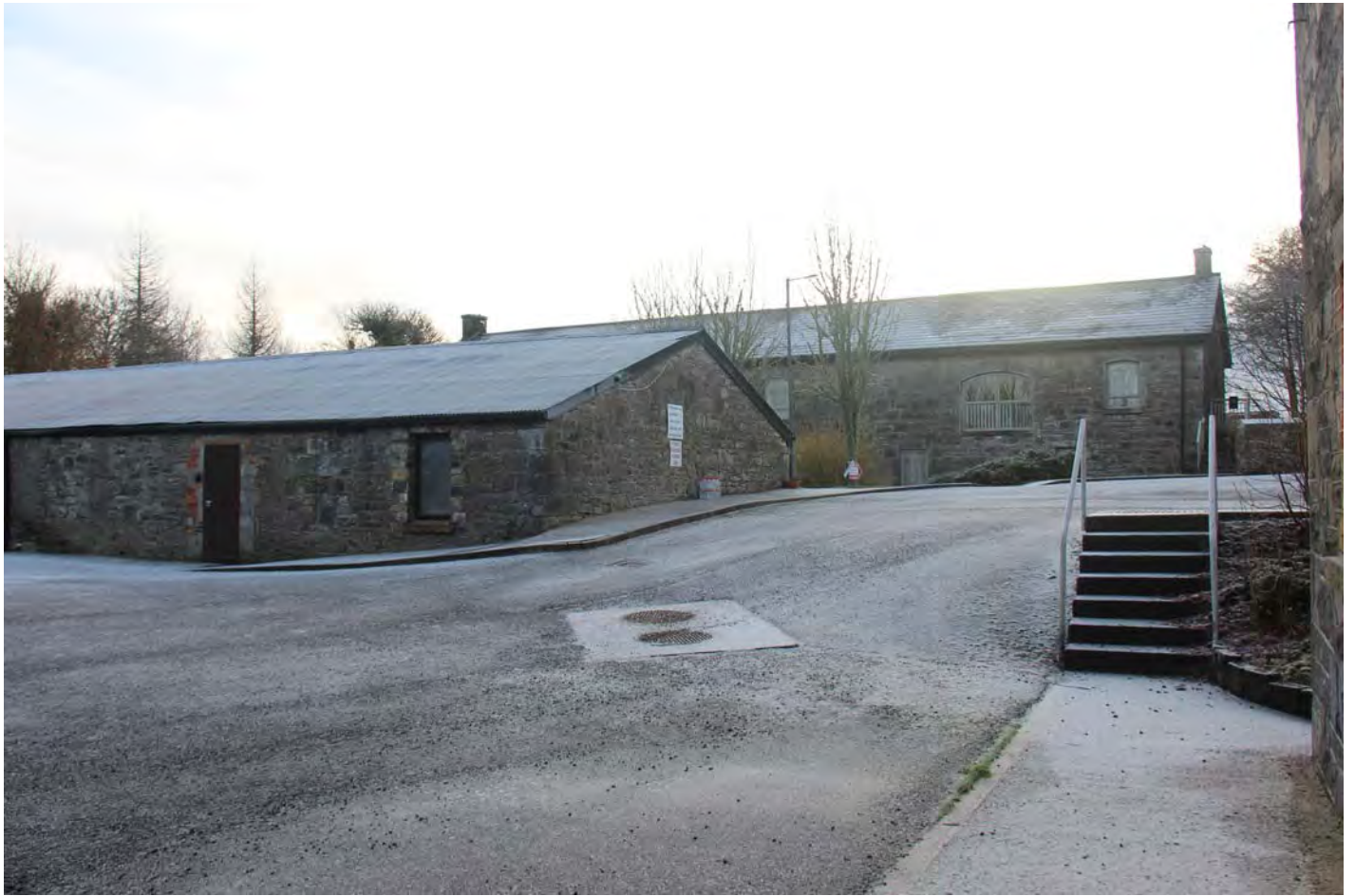
J991_P07 View of North Elevations of Fromer Outbuilding
