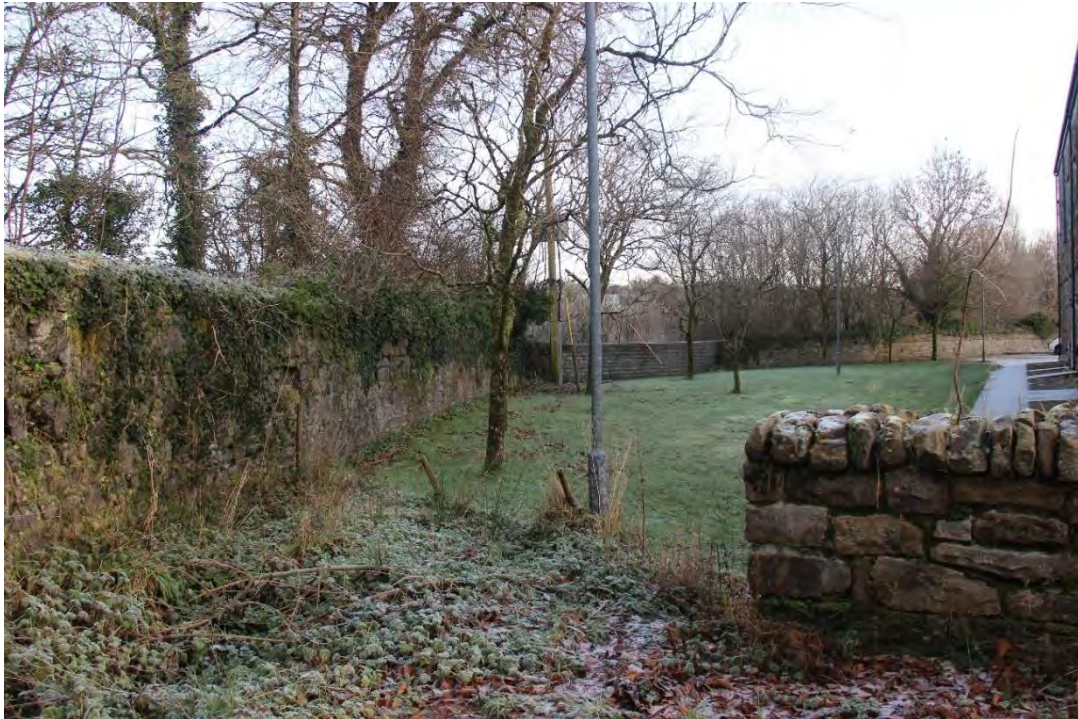
Photograph 6 - Existing Boundary Wall
