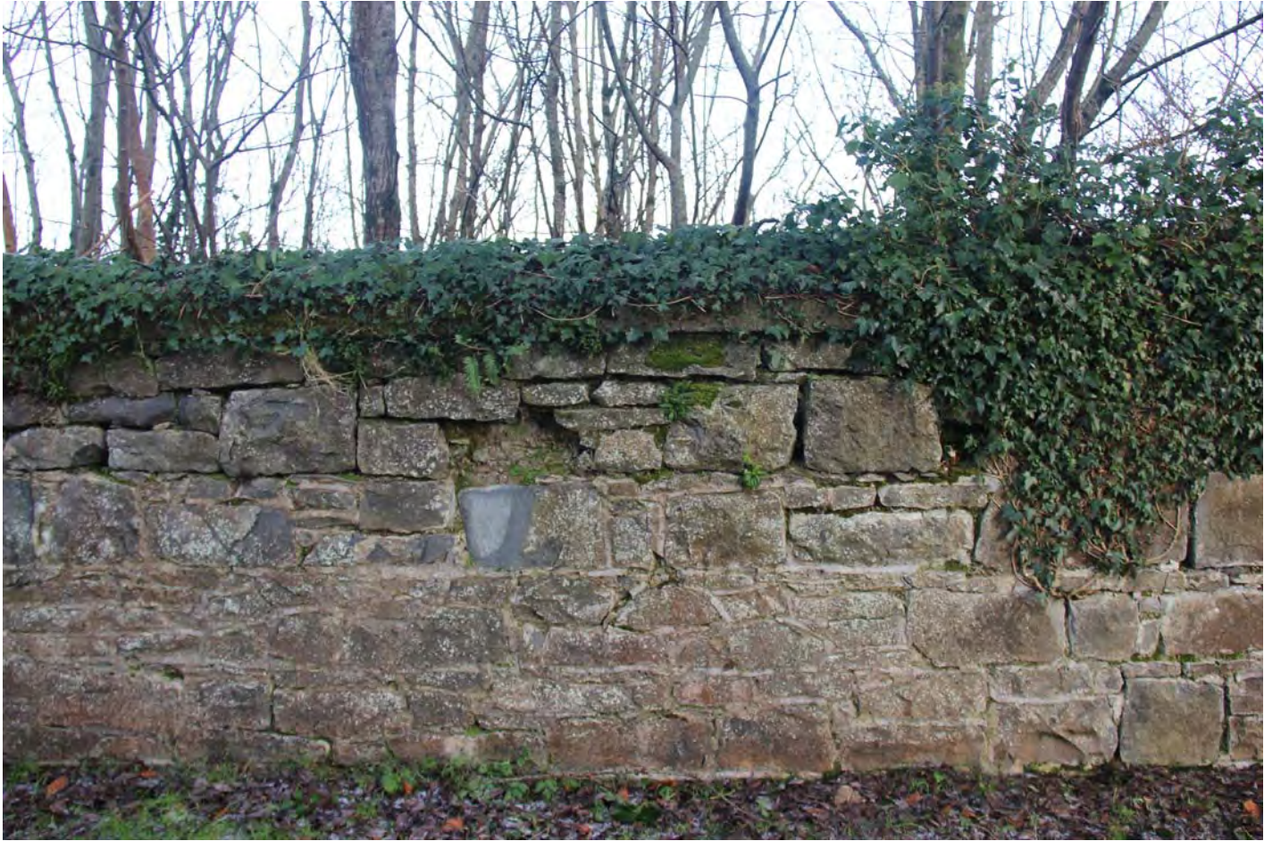
J991_P11 Existing Boundary Wall Section B1
