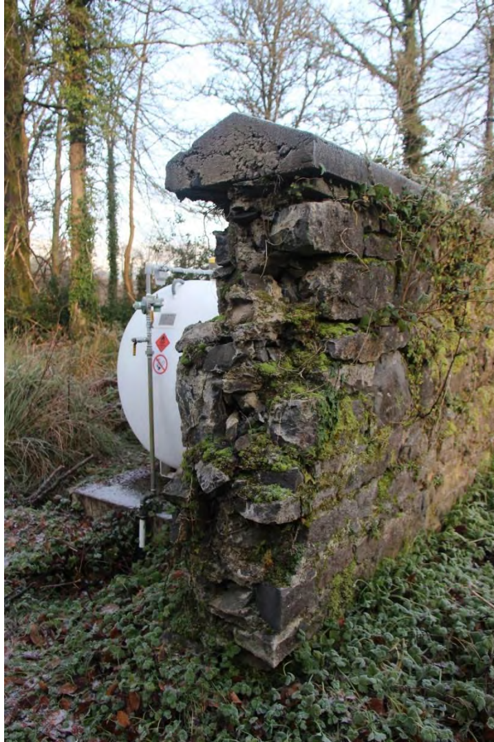
Photograph 15 - Section D Eastern side of gap in Boundary Wall
