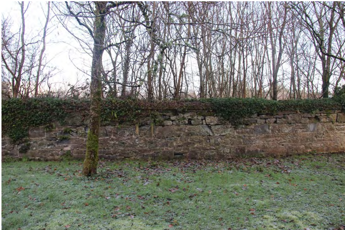
J991_P13 Existing Boundary Wall Section B1
