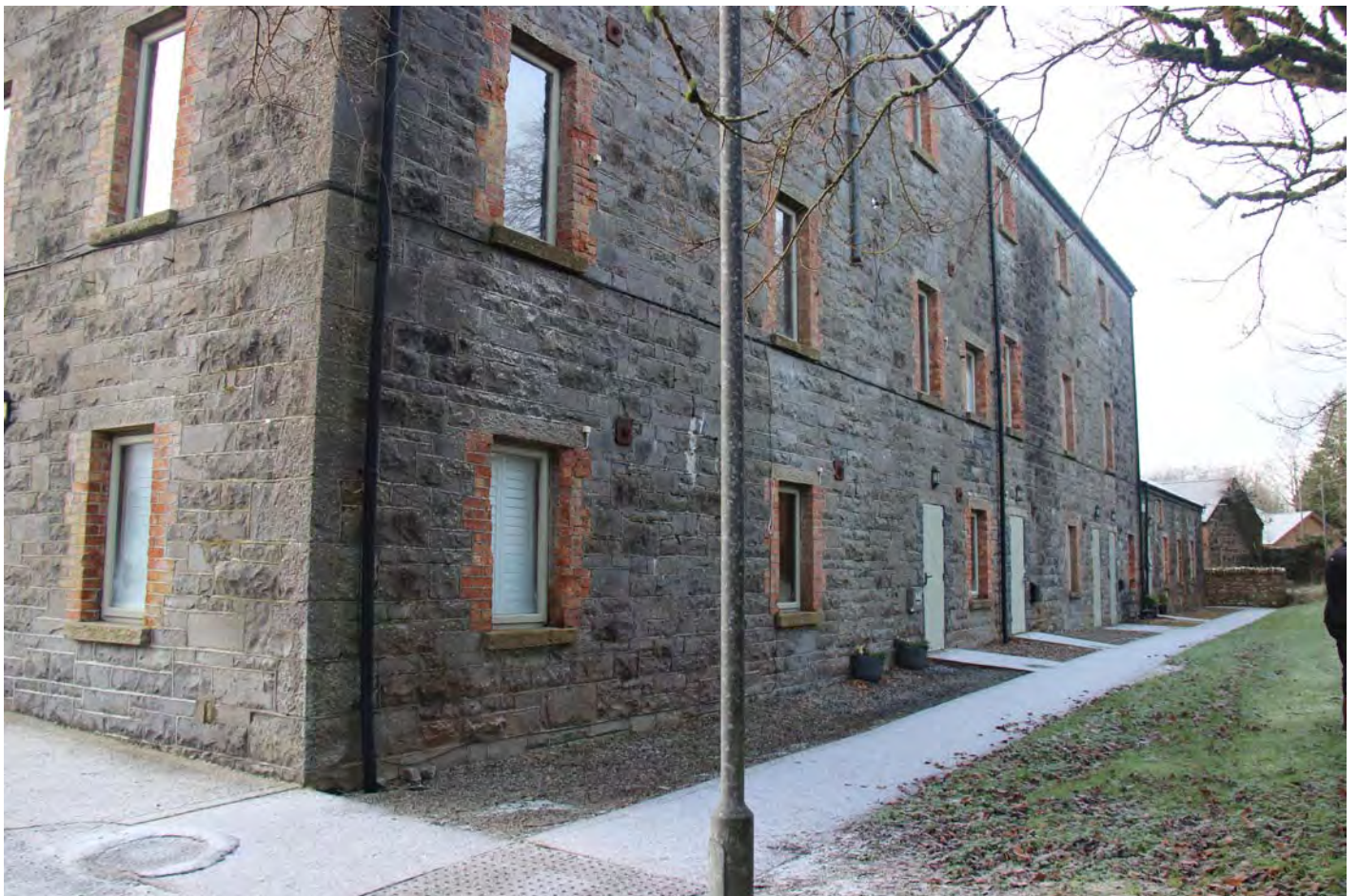
J991_P08 View of North Elevation of The Mill Apartments
