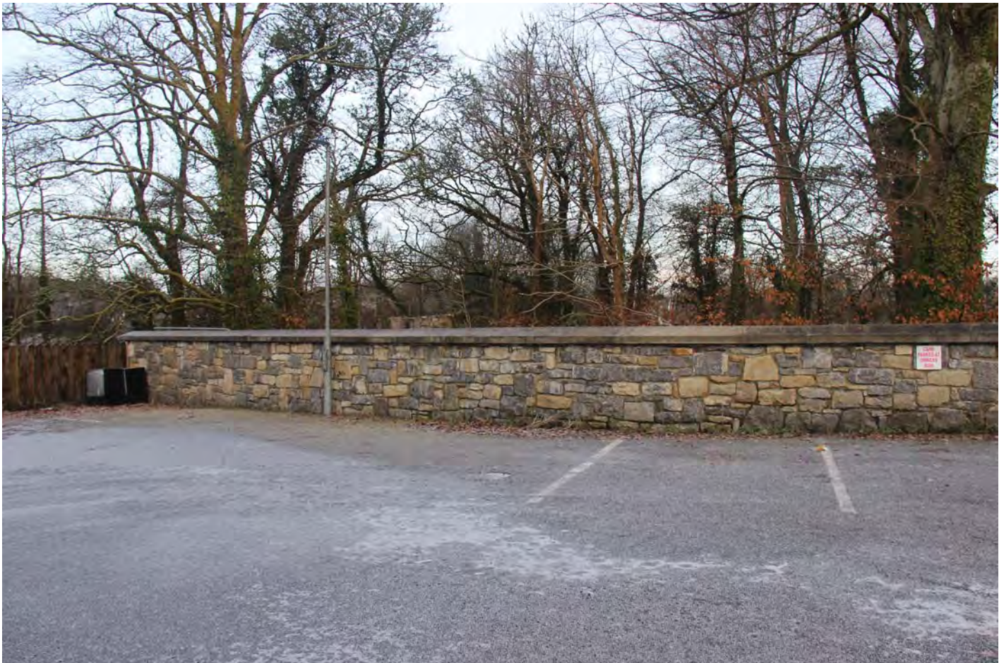
J991_P22 Existing Boundary Wall Section E
