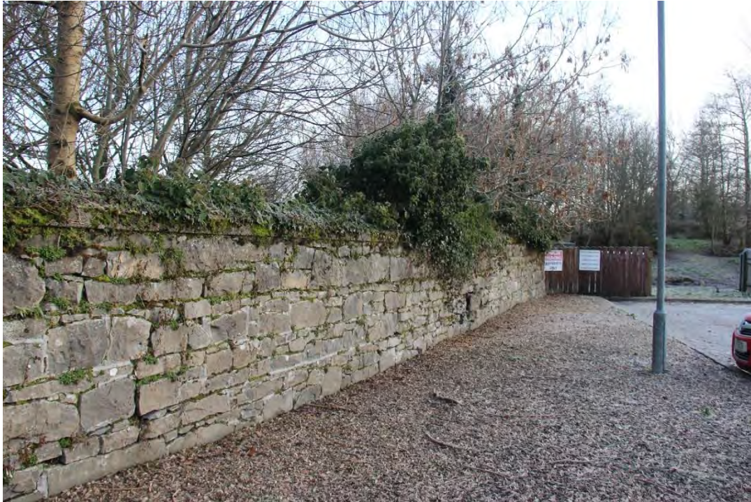
Photograph 9 - Section B Original Boundary Wall with Concrete Capping
