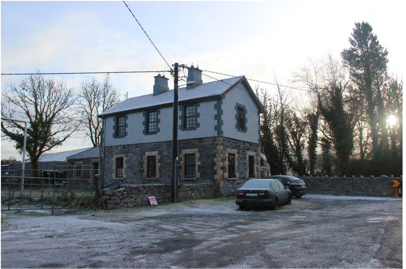
J991_P27 View of Northern and Western Elevations of Former Station House
