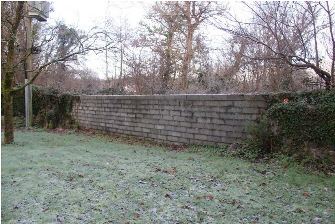
Photograph 13 - Section C Modern Blockwork Wall
