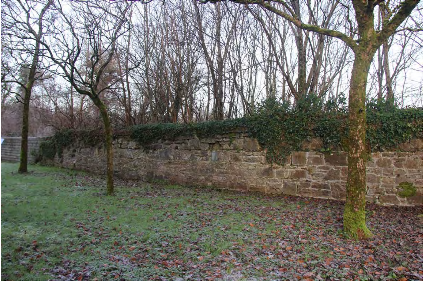
J991_P09 Existing Boundary Wall Section B to Section C
