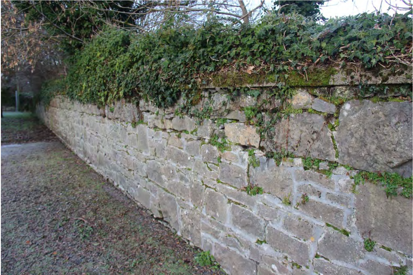
J991_P04 Existing Boundary Wall Section B
