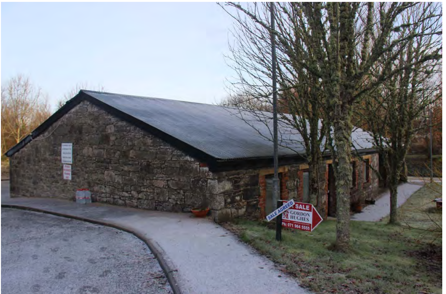
J991_P36 View of Northern and Western Elevations of Former Outbuildings
