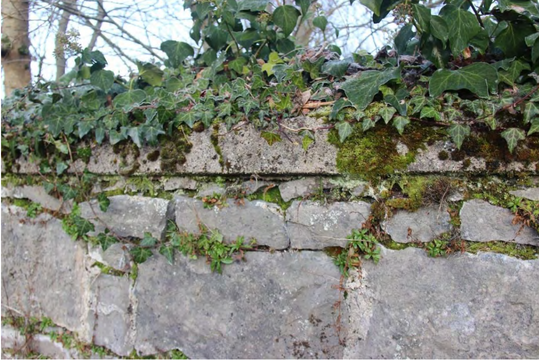
Photograph 10 - Section B Detail of Concrete Capping
