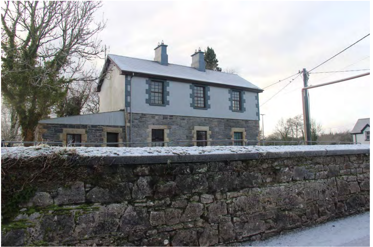
J991_P29 View of Northern Elevation of Former Station House
