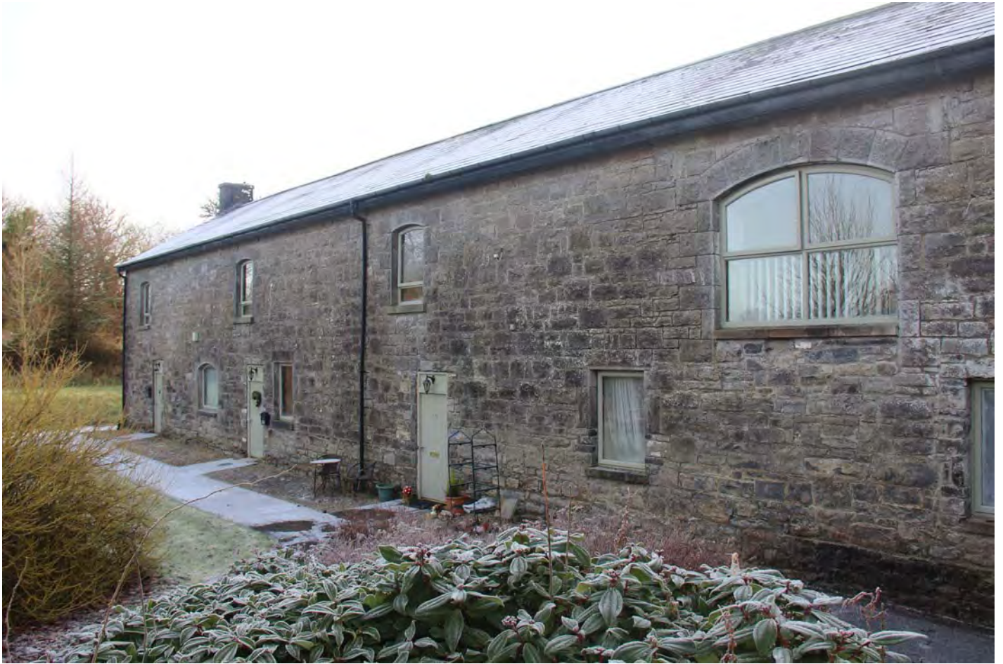
J991_P35 View of Northern Elevation of Former Outbuildings
