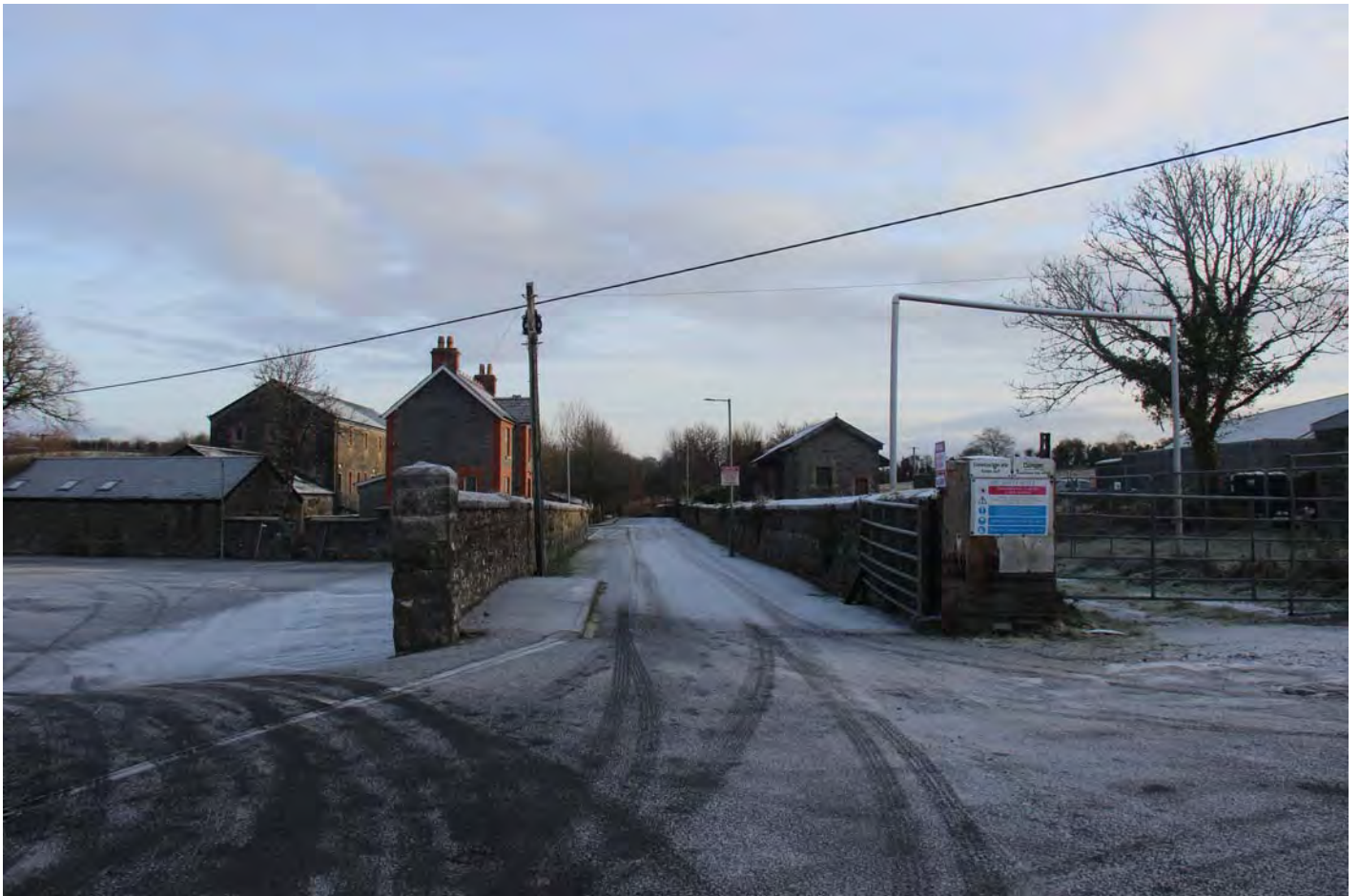
J991_P26 View of Entrance to Former Dromahair Railway Station
