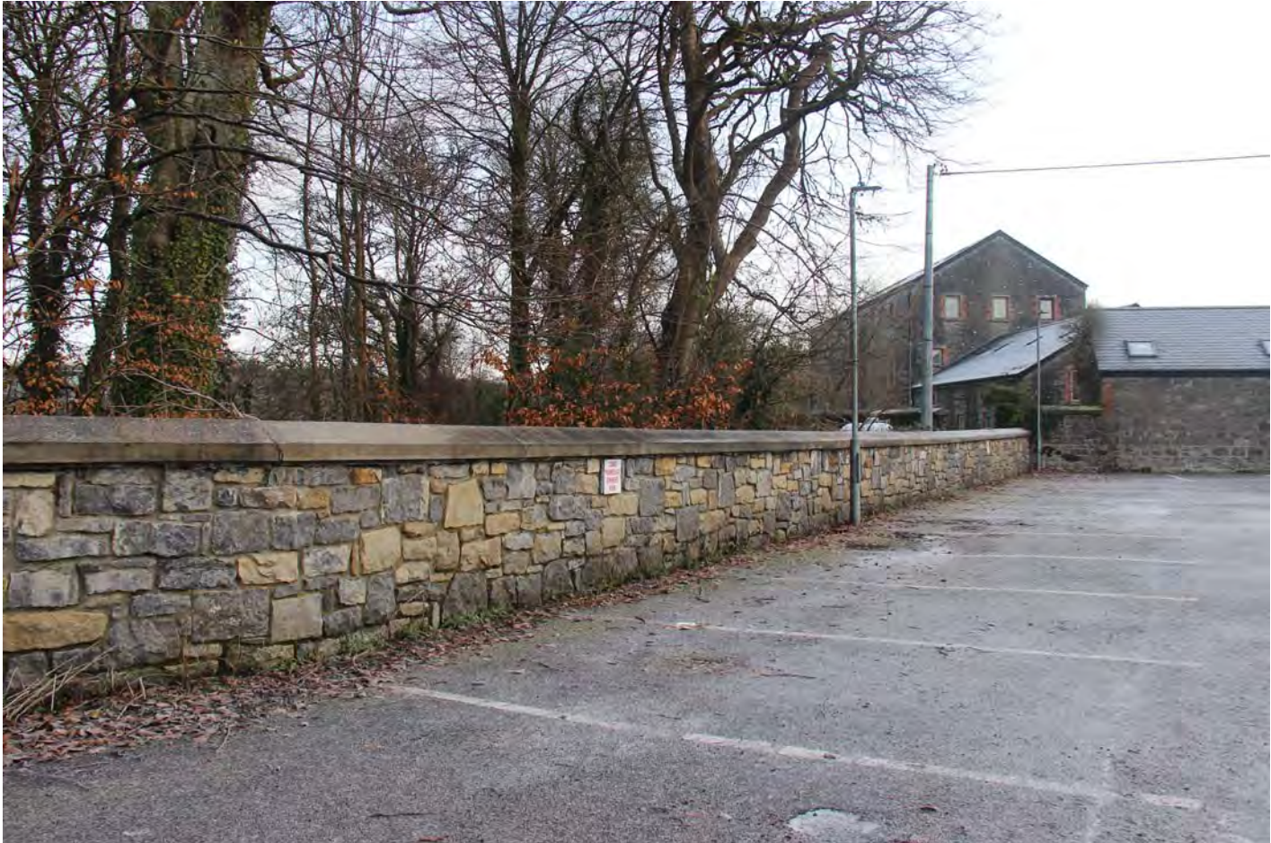
J991_P21 Existing Boundary Wall Section E
