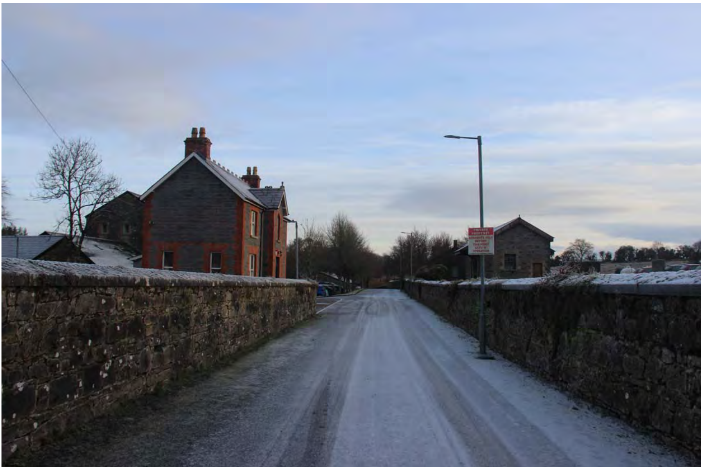
J991_P28 View of Entrance to Former Dromahair Railway Station
