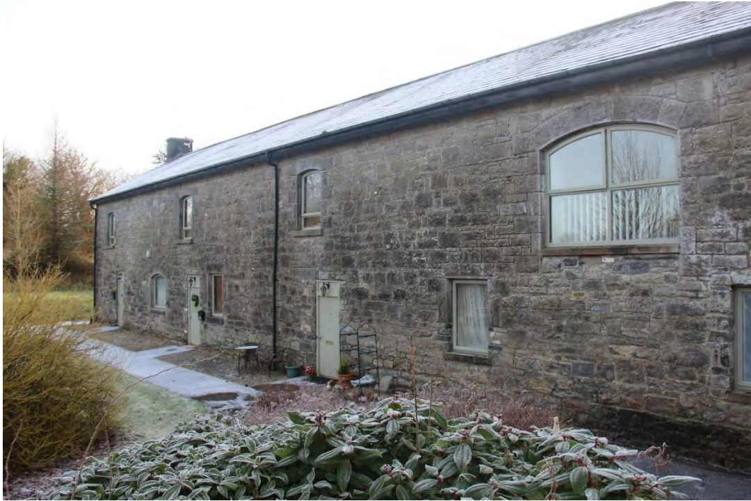
Photograph 3 - Apartments, Former Goods Shed & Outbuilding, Dromahair Railway Station (RPS 70)
