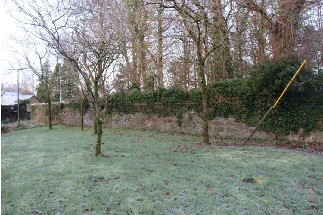
Photograph 14 - Section D Original Boundary Wall with Concrete Capping
