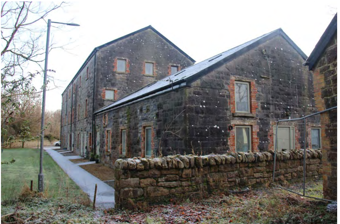
J991_P18 View of Western Elevation of The Mill Apartments
