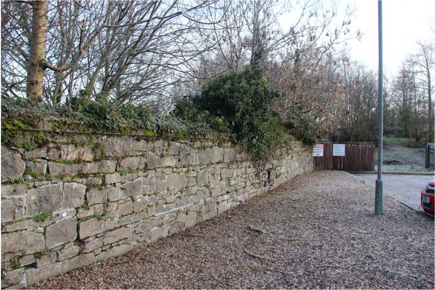
J991_P05 Existing Boundary Wall Section B
