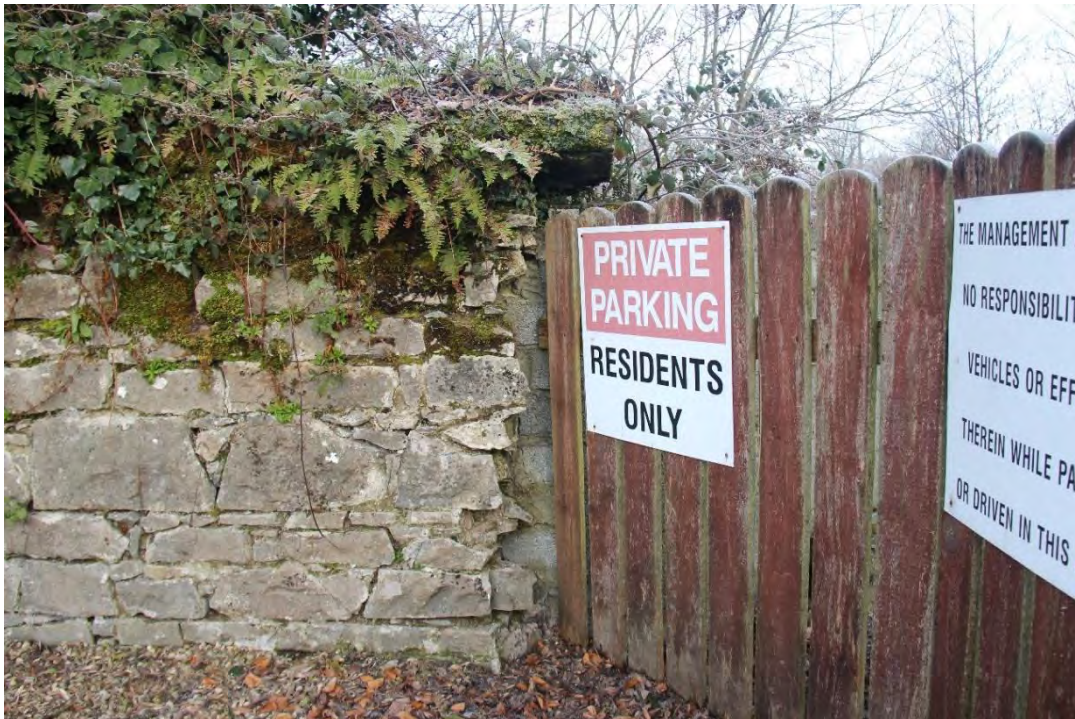
Photograph 8 - Section A Modern Blockwork joining Section B Original Boundary Wall
