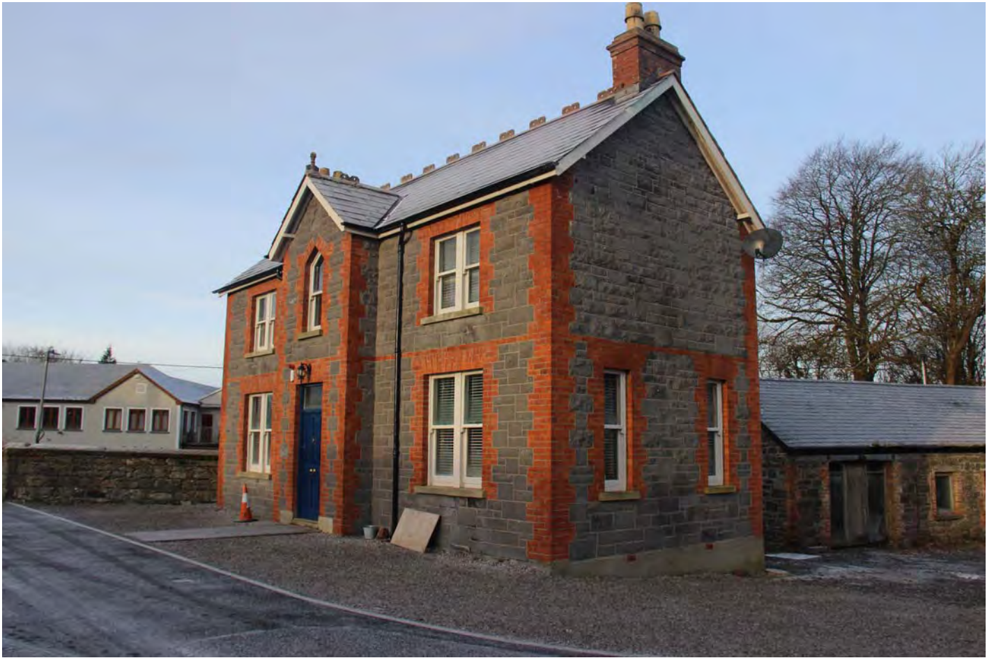
J991_P31 View of Southern and Eastern Elevations of Former Station Masters House
