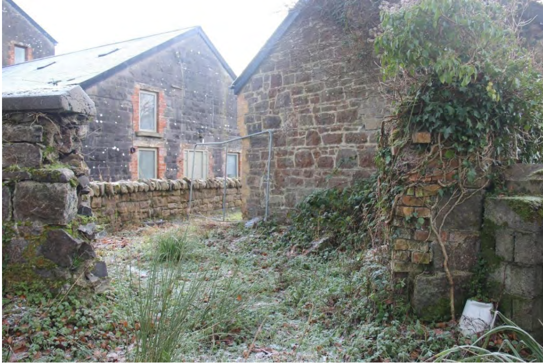
Photograph 16 - Section D Detail of Gap in section with brick edged opening to right (Western Side)
