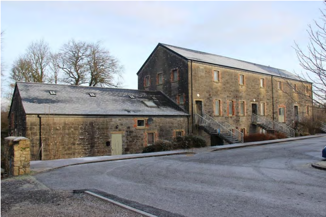
Photograph 2 - The Mill Apartments, Former Railway Warehouse & Outbuilding, Dromahair Railway Station (RPS 71)
