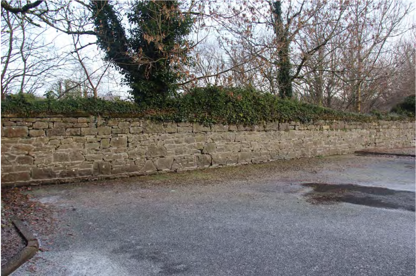
J991_P06 Existing Boundary Wall Section B
