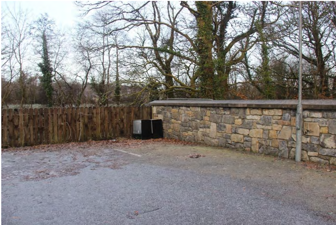
Photograph 18 - Section F Timber Fence joining Section E Modern Wall
