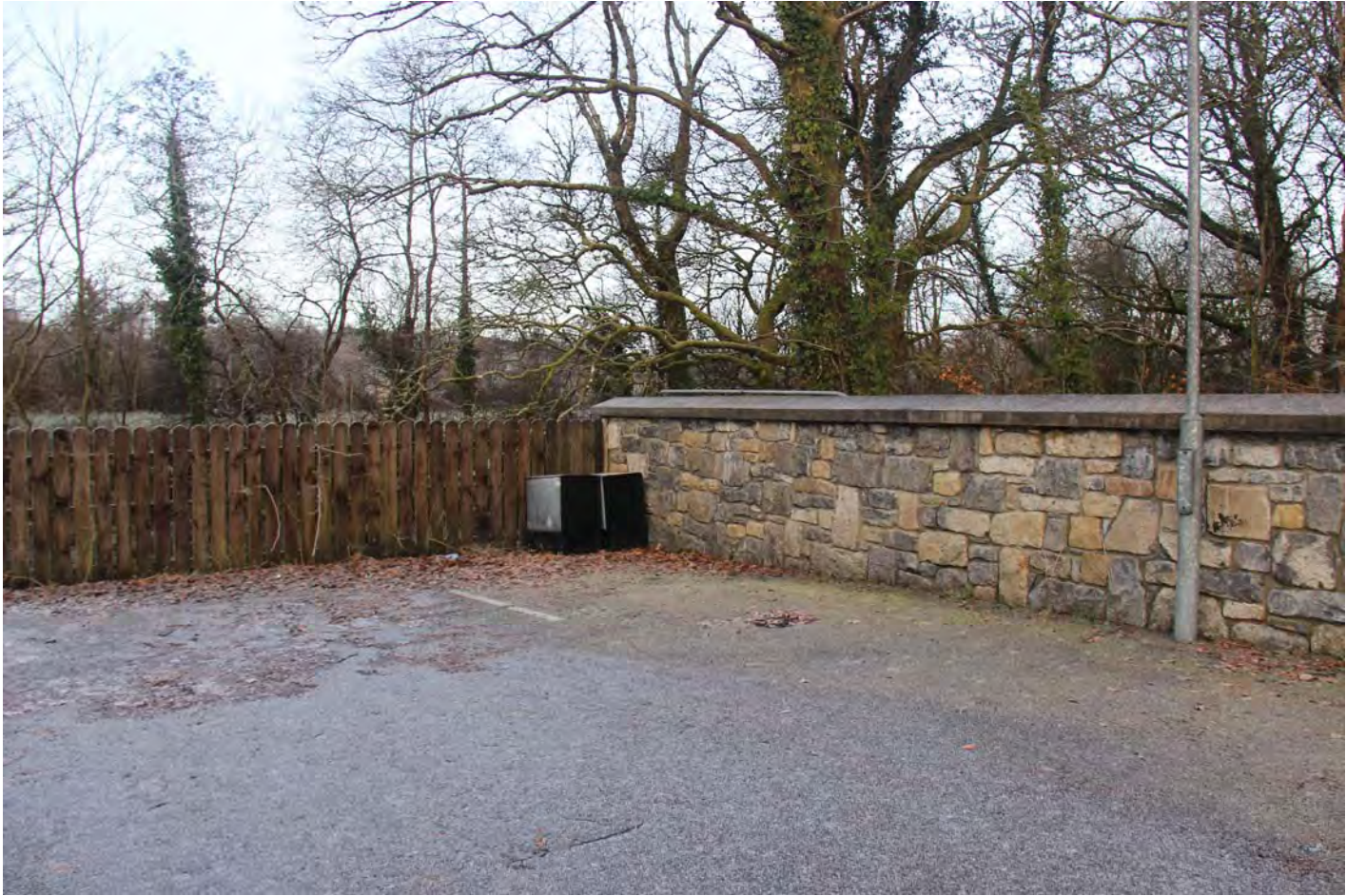
J991_P23 Existing Boundary Wall Section E
