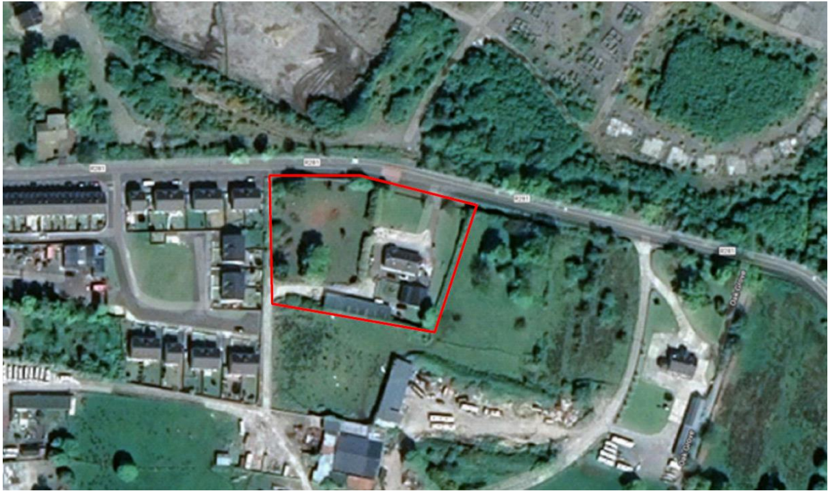
Figure 3 Satellite view of the land in Kinlough
