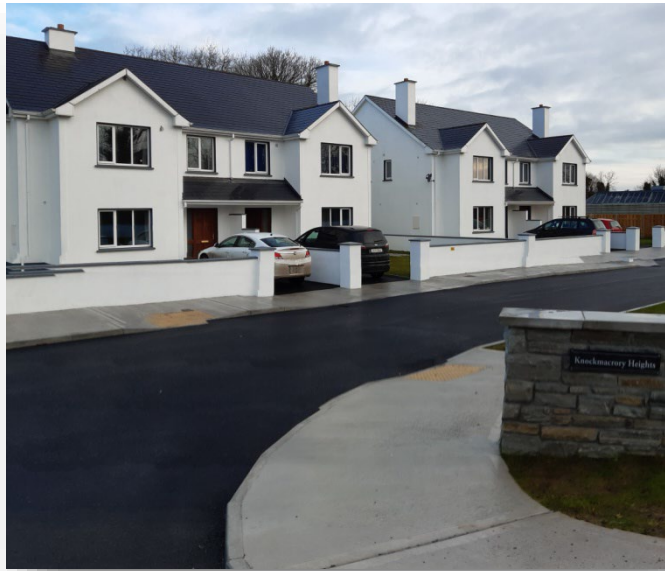
Figure 2: Completion of Knockmacrory Heights, Roosky – A Local Authority Turn Key Development
