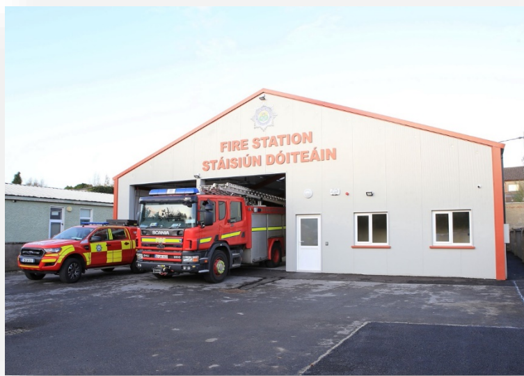
Figure 14: New Fire Station Building in Ballinamore
