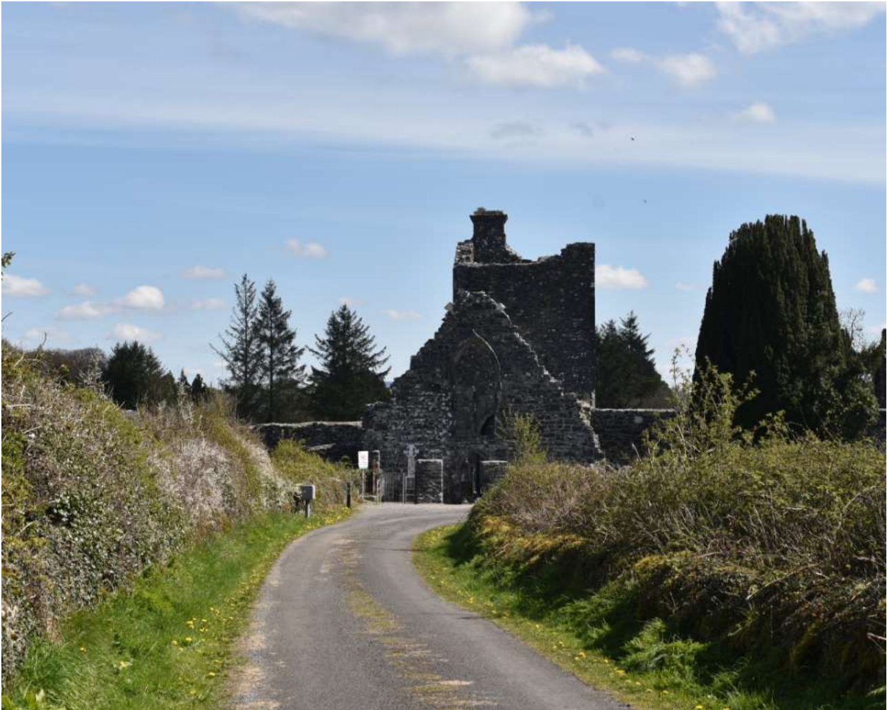
The siting and design of commercial forestry needs to have regard for the landscape setting of important heritage assets including Creevelea Abbey.
