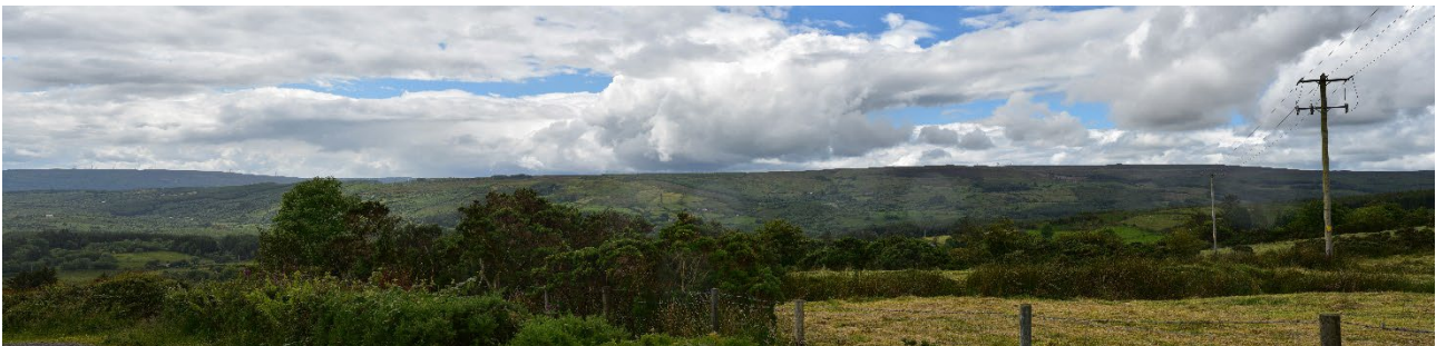
Plate 8-1 Moorland Hills in the Boleybrack Mountain LCA - a landscape comprised of smooth rolling hills and featuring existing wind turbines and commercial forestry.
