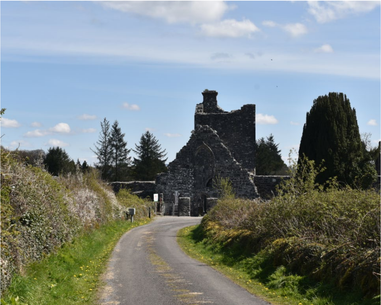
The siting and design of commercial coniferous forestry needs to have regard for the landscape setting of important heritage assets including Creevelea Abbey.
