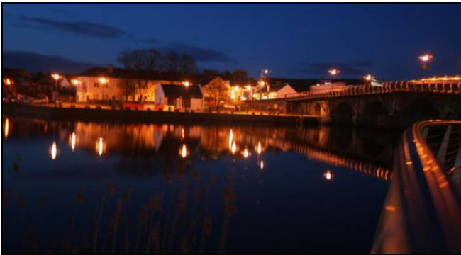
Photo 2.6b Night View of Recently Completed Footbridge
