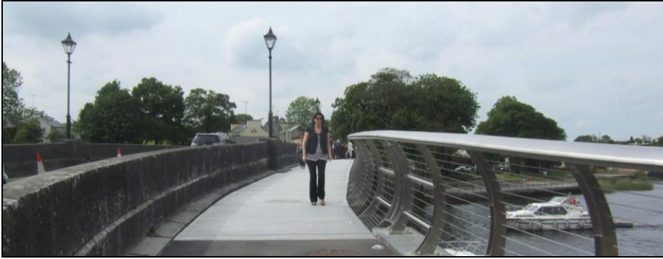
Photo 2.6a Recently Completed Footbridge
