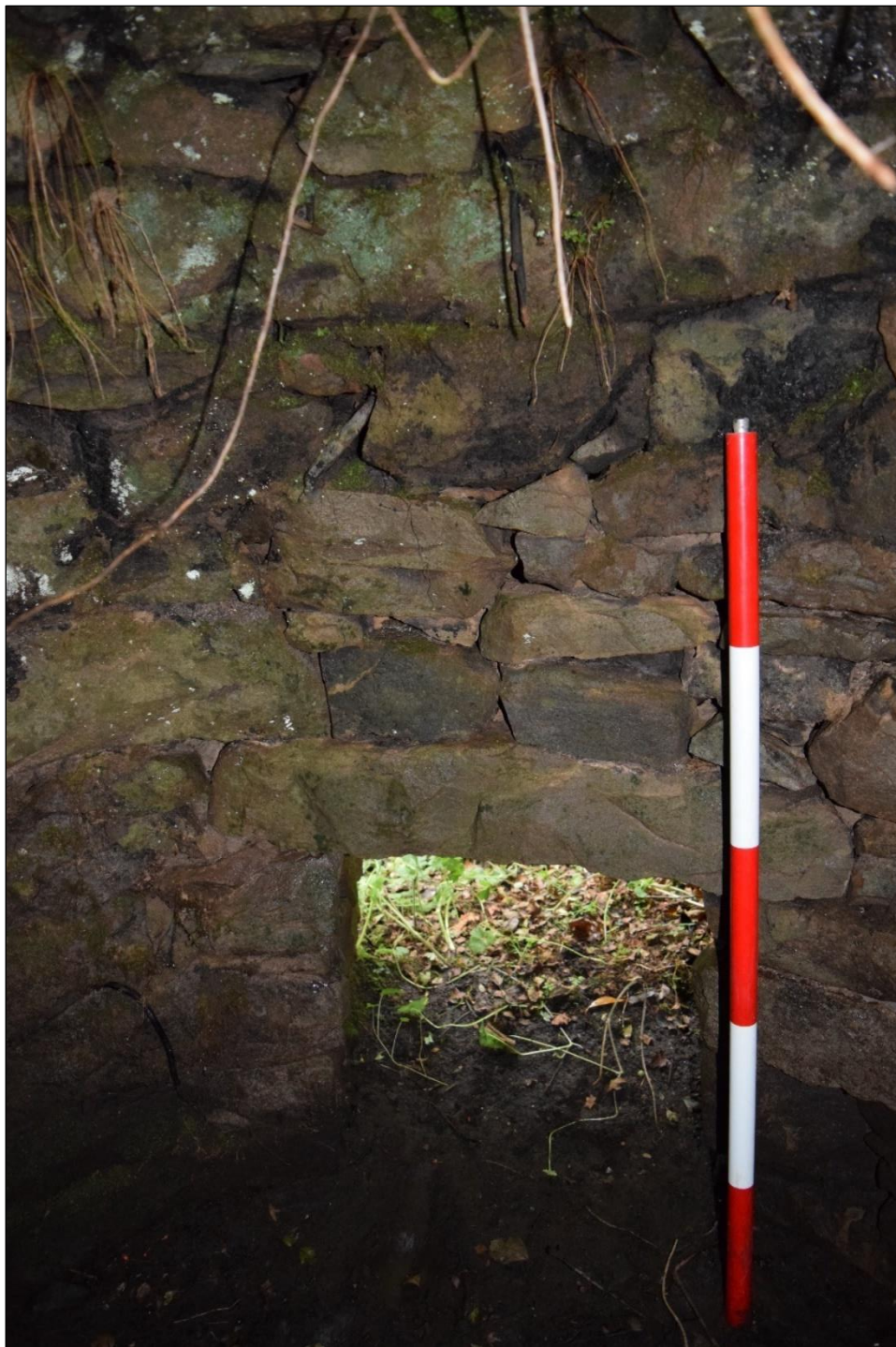
Plate 10: Interior of Killadiskert Sweathouse (LE018-062----)
