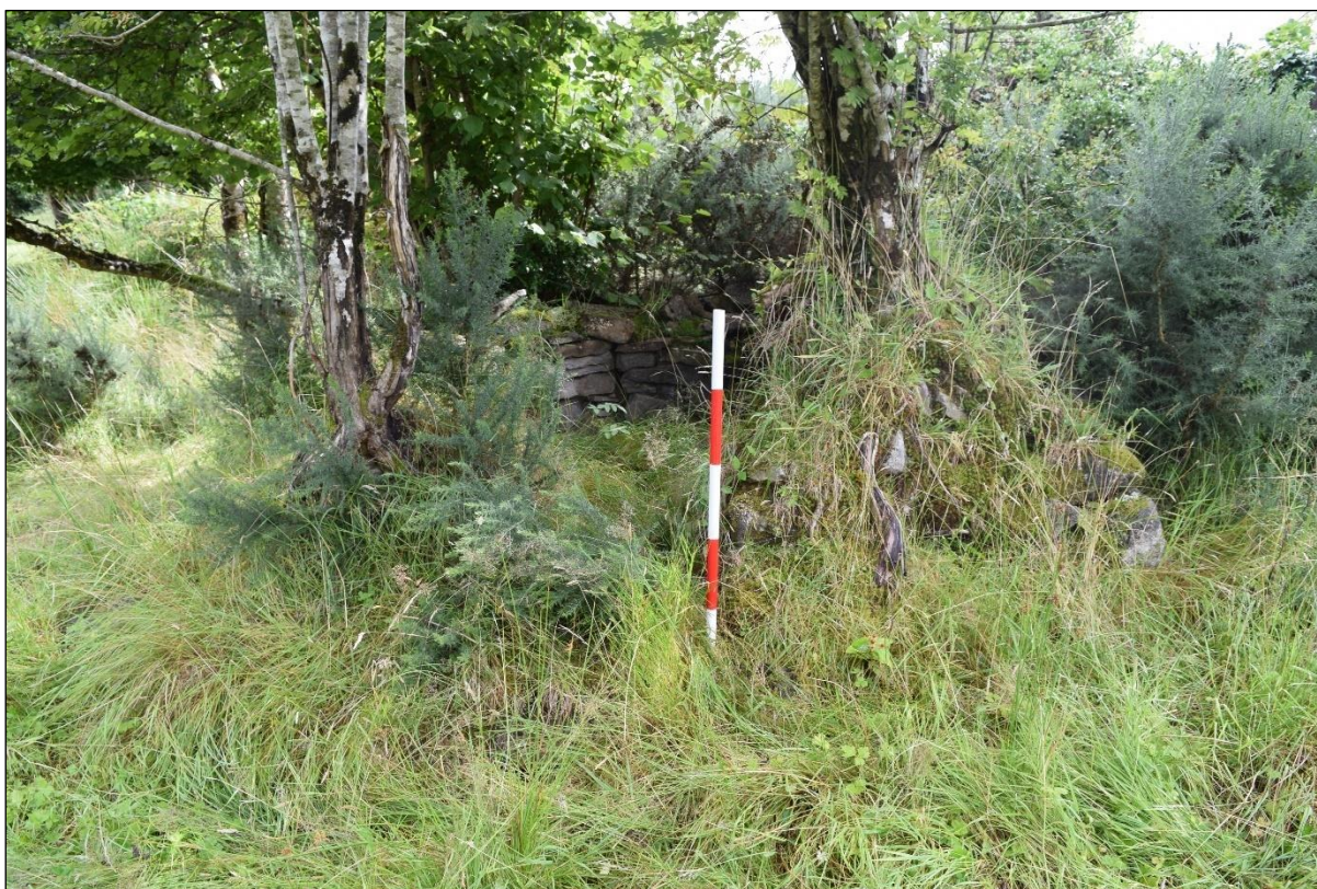
Plate 12: A previously unrecorded Sweathouse at Cloone, Kinlough, now collapsed with trees growing from the mound
