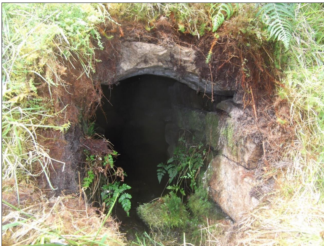
Plate 9: Entrance with curved lintel at Greaghmagloach LE016-024---- (photo by D. McCarthy)
