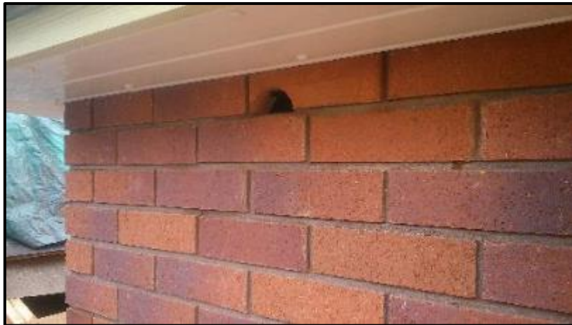
Figure 15: A Swift Brick installed in a newly erected redbrick wall. Photo: www.birdbrickhouses.co.uk
