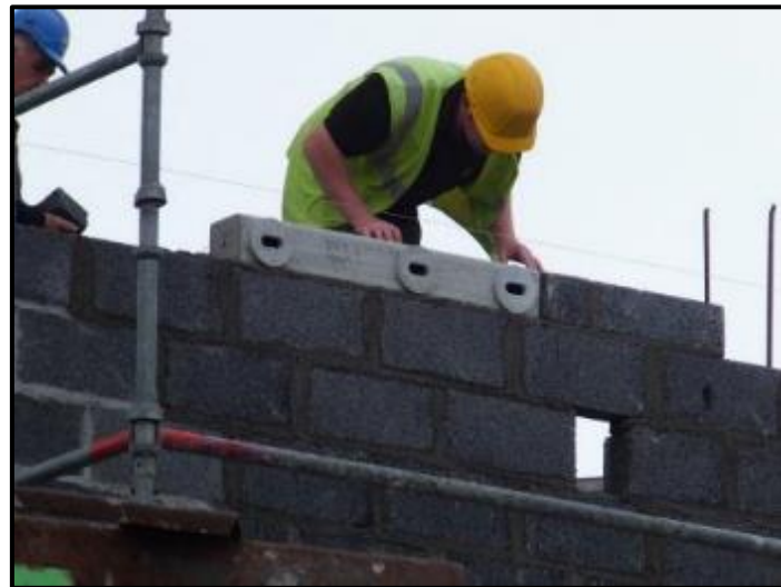
Figure 13: Installing Swift boxes as part of the fabric of the wall. Photo: Lynda Huxley
