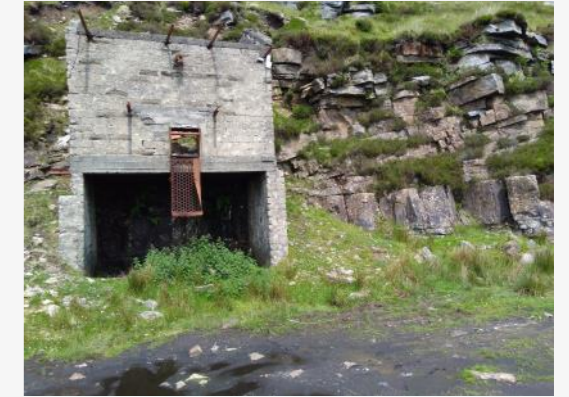
Screening plant with cross-bedded sandstone strata on the right.
