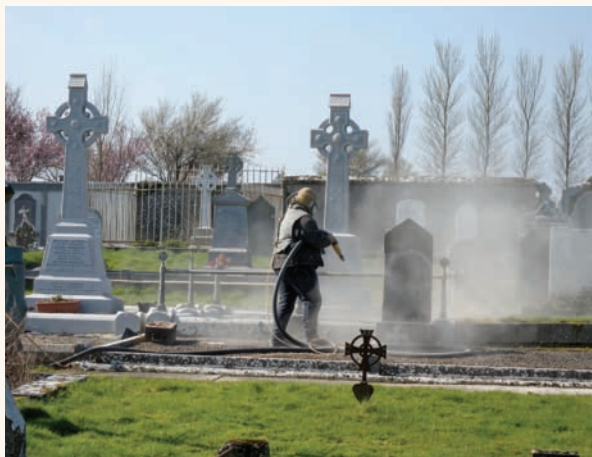
The sandblasting of memorials speeds up the process of decay of stone and should be avoided
