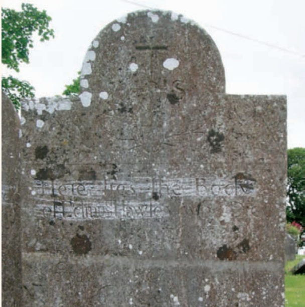
An overly heavy chalk rubbing of a memorial inscription can cause damage
