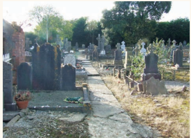
A deteriorating concrete pathway which will require maintenance works
