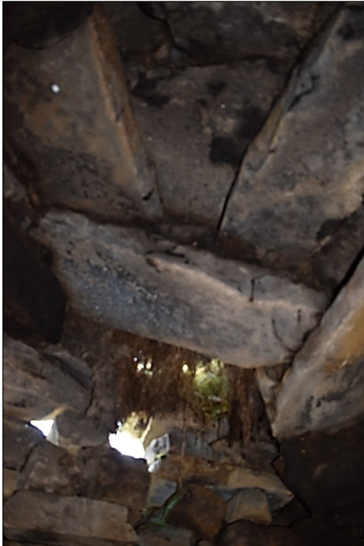
Plate 10: Front part of ceiling at Kiltyclogher 2
