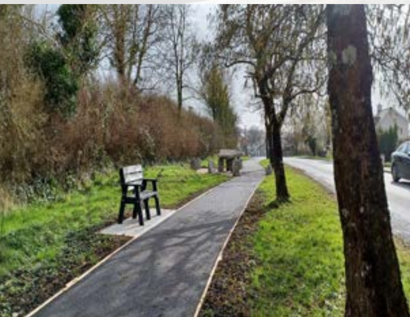
Completed Active Travel Scheme at Leitrim Village
