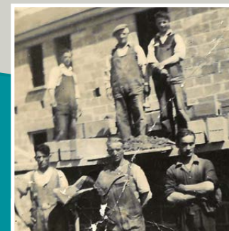
Roads, Housing, Motoring & Emergency Services
